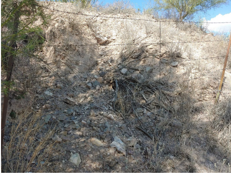
Figure 69. Additional Strand of Wire Beneath a Four-Strand ROW Fence
