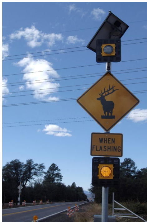
Figure 79. Elk Crossing Alert Signage Triggered by a Detection System at an Elk Crosswalk
