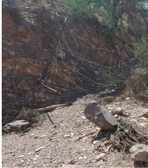
Figure 61. Raised Bottom Wire Access Point Where Fence Enters a Wash
