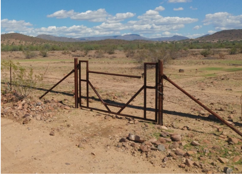
Figure 65. Equestrian Gate with an Aperture Allowing Burro Passage
