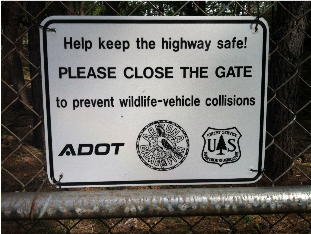
Figure 76. Sign to Reduce the Incidence of Unclosed Gates
