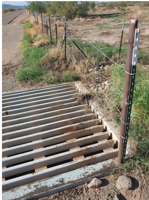
Figure 72. Wing Fence at a Crossing Guard Tie-In
