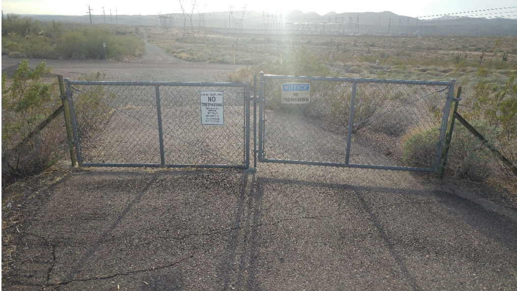
Figure 74. ADOT Type 1 Double Gate
