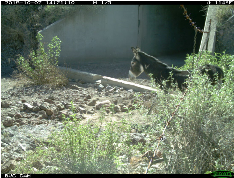
Figure 41. Burro Leaving an ROW Through a Raised Bottom Wire Adjacent to a Below-Grade Crossing Structure
