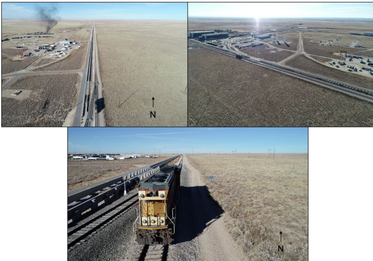
Figure 2. Aerial views of the Precision Test Track at TTC
