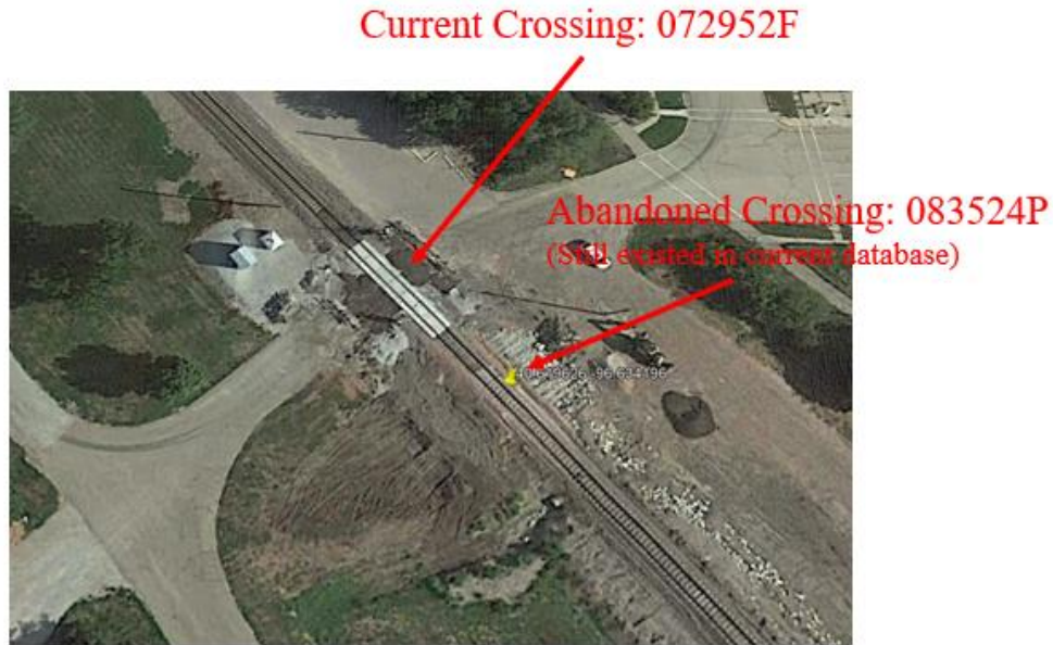
Figure 4.4 An Example of an Abandoned Crossing (083524P)
