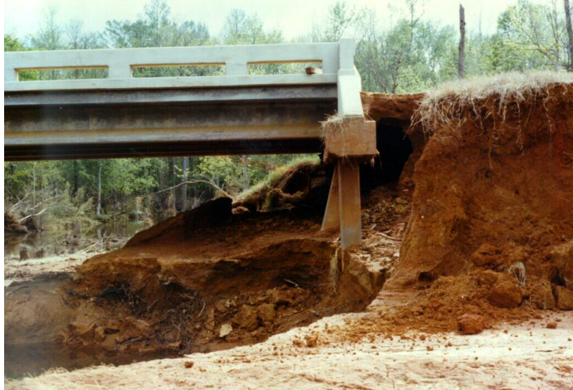
Figure 1. Abutment scour at a bridge approach
