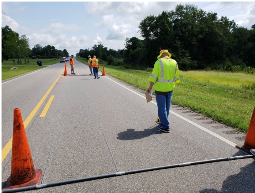
Figure 14. Example of a template used to define the wheel path areas surveyed.
