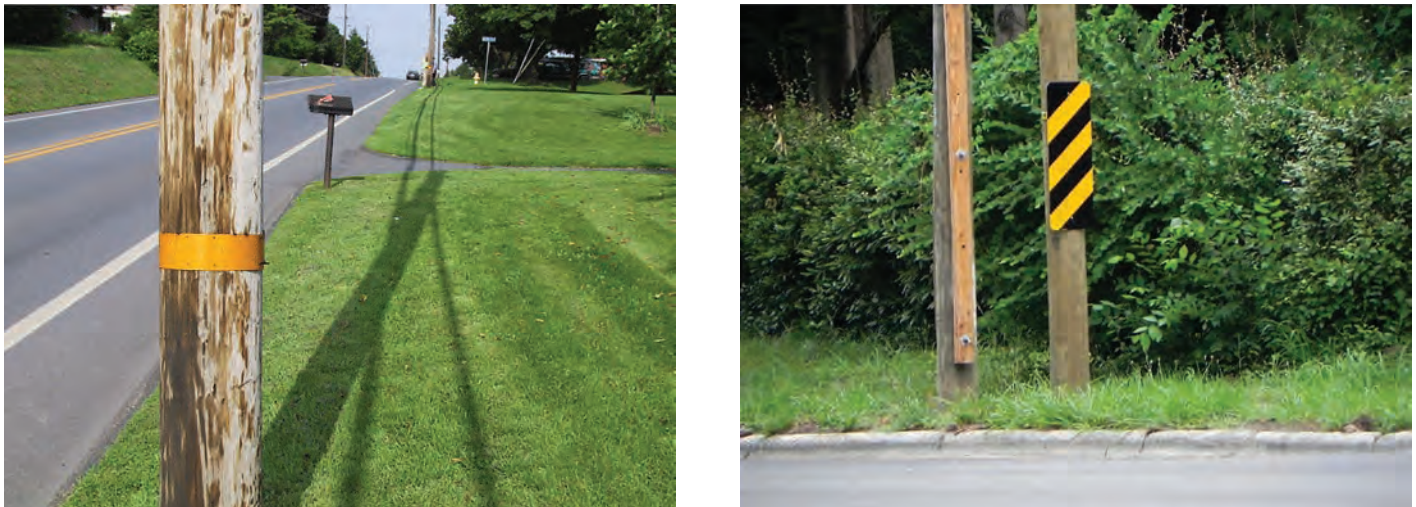
Figure 27. Examples of reflective tape on utility pole (left) and reflective panel (right) (Photos: Kevin Zegeer).
