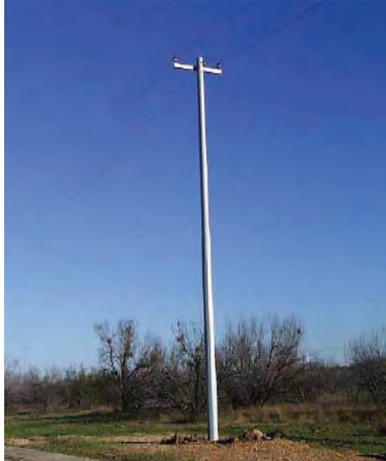
Figure 23. Example of a composite breakaway utility pole (Foedinger et al. 2003).
