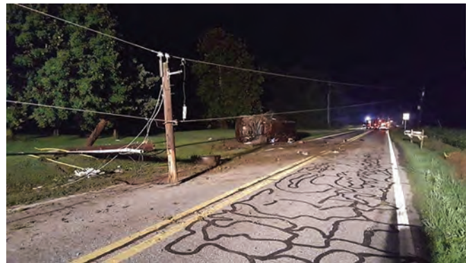
Figure 16. High-risk poles along a tangent section (Image: Delaware DOT).
