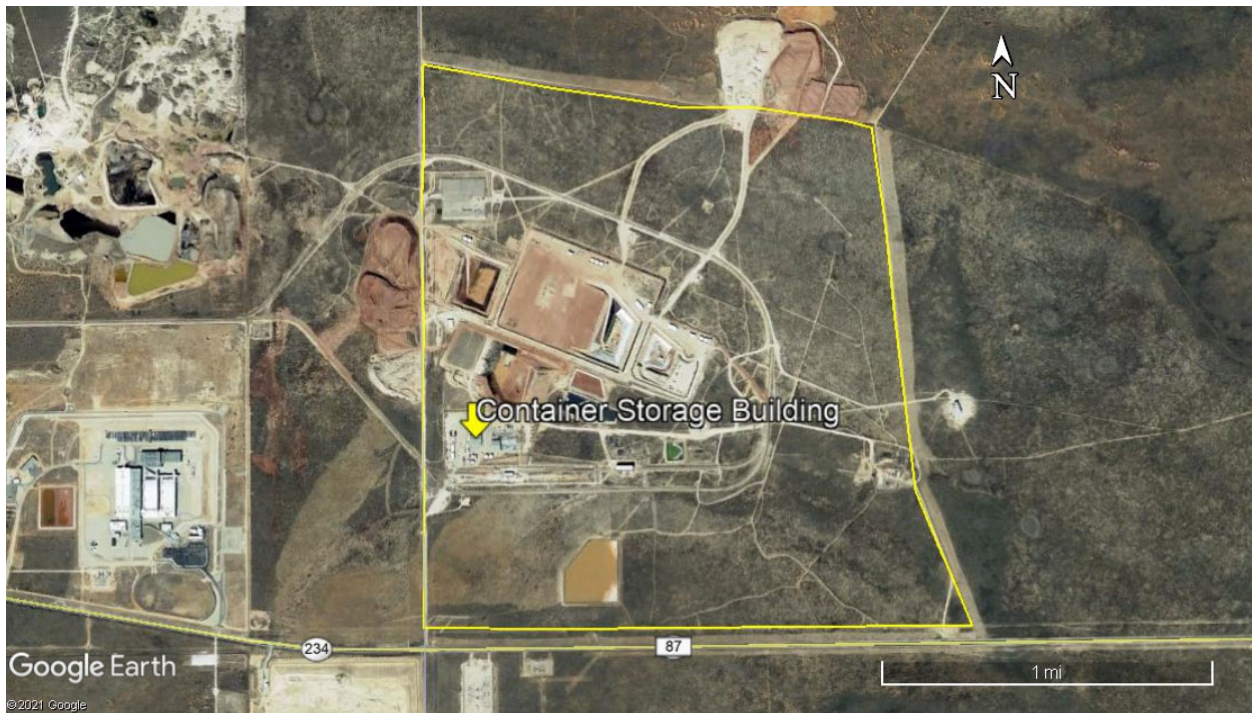
Figure 3-2 Aerial View of WCS Container Storage Building
