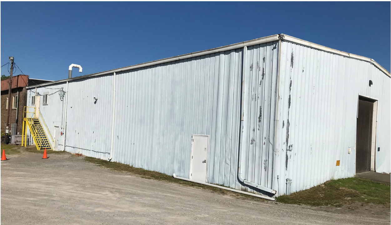
Figure 2-13 Storage Warehouse Building at the Clean Harbors Greenbrier Site
