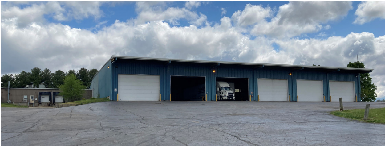
Figure 2-14 CSB-2 (foreground) and CSB-1 (rear left) at the Clean Harbors Pecatonica Site
