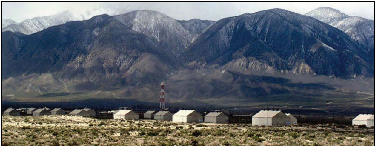
Figure 2-3 Existing Storage Buildings at the HWAD in Nevada
