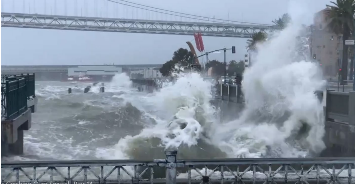
Figure A-5: Overtopping of Seawall in March 2023
