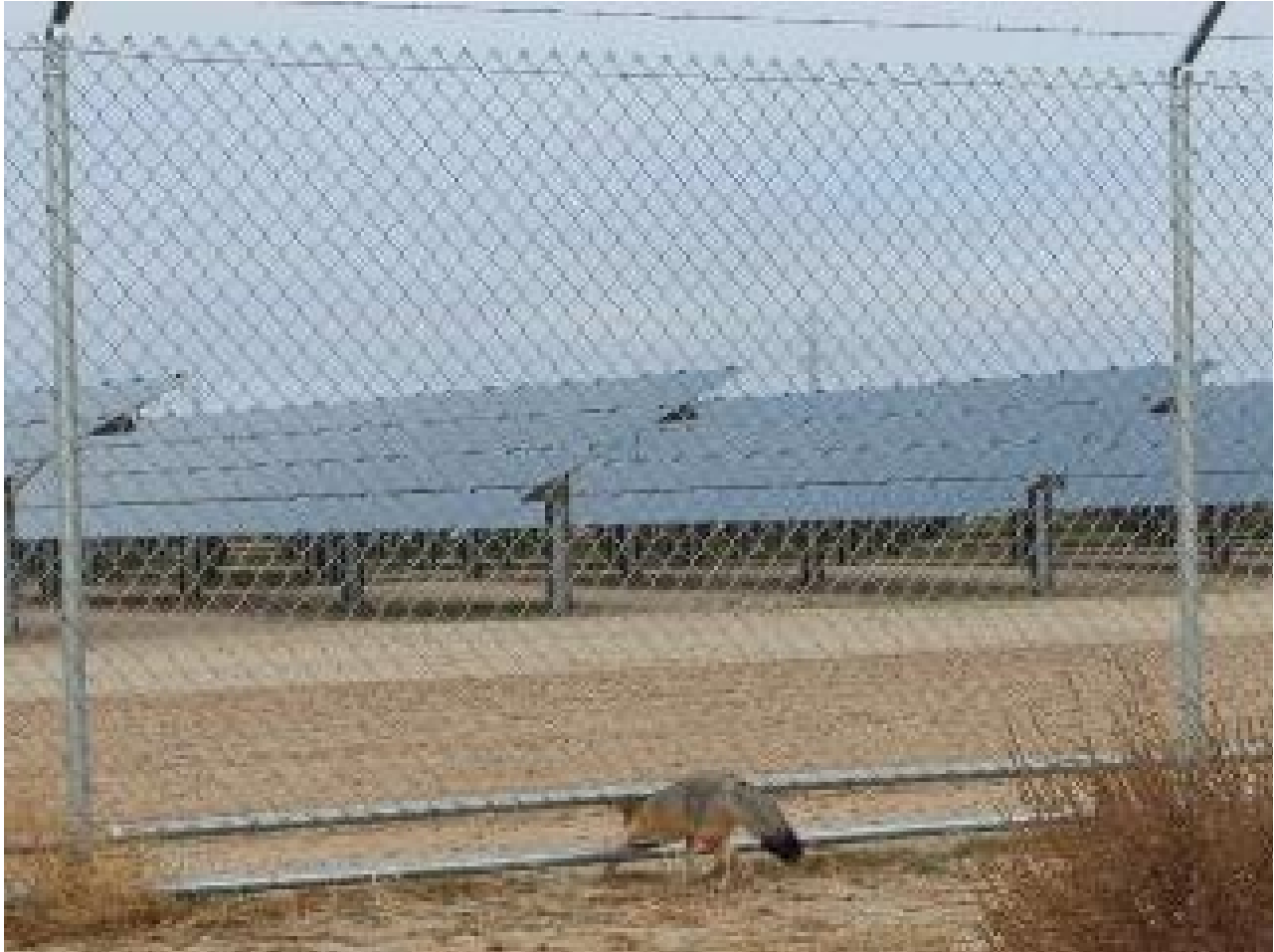
Figure 2.2-1 Example of Small Mammal Permeable Fencing
