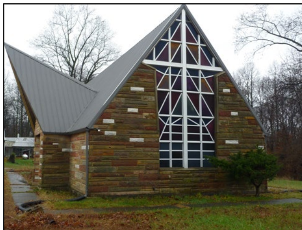
FIGURE 31. BRINEGAR CHAPEL PHOTOGRAPH (C. 2011)
