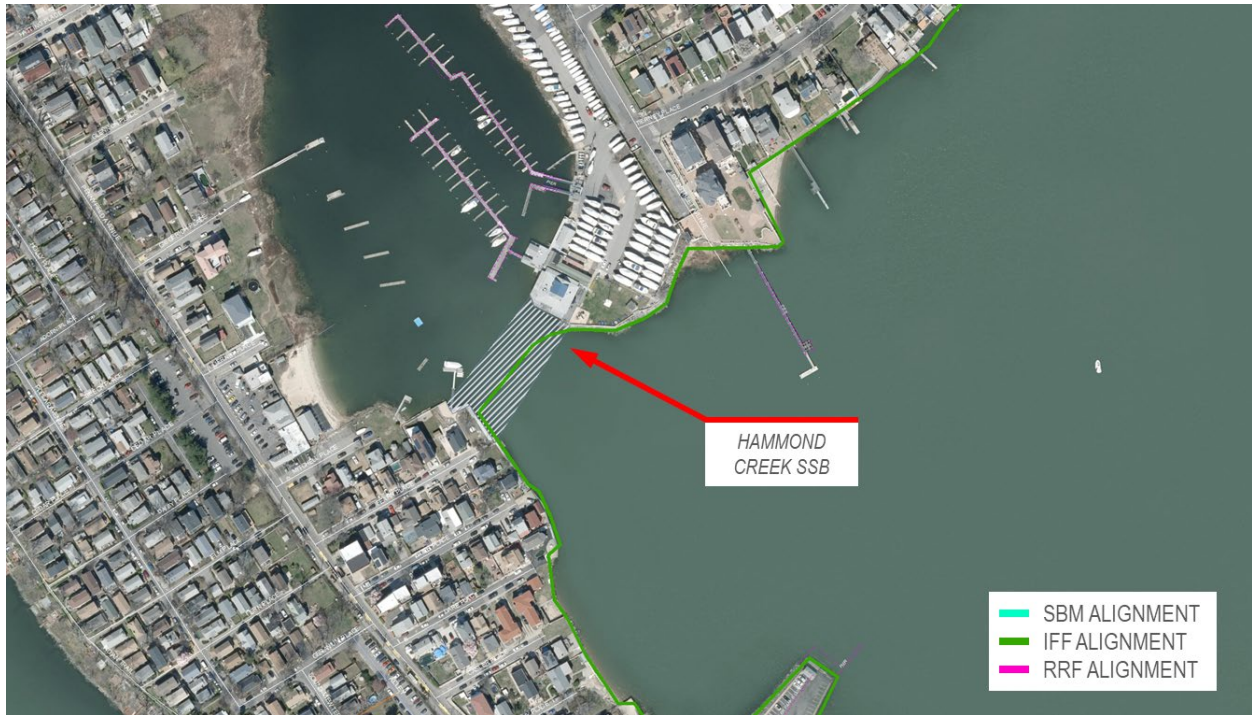
Figure 6-32: Hammond Creek Storm Surge Barrier Approximate Location
