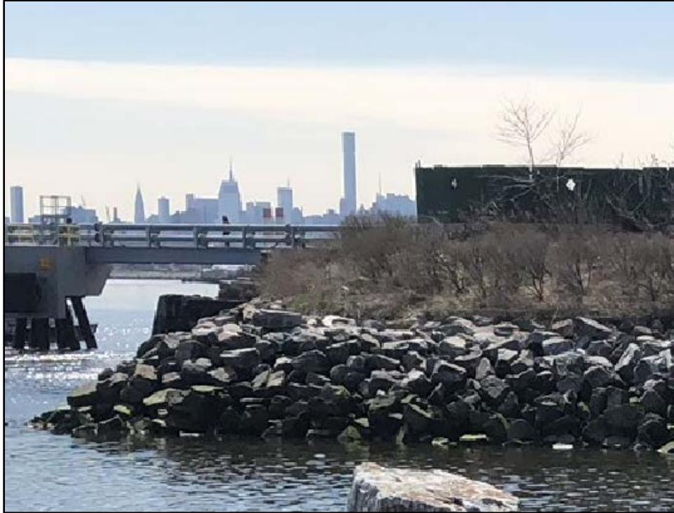
Figure 3-10: Rubble Mound Structure in Bronx, New York (M&N, 2017)
