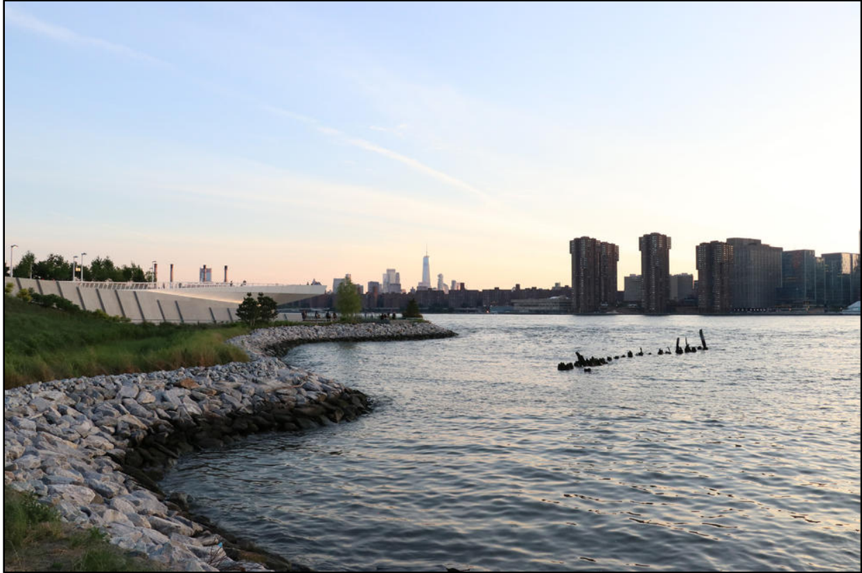
Figure 3-32: Revetment at Hunters Point, NY (photo credit: Nicole Avella)
