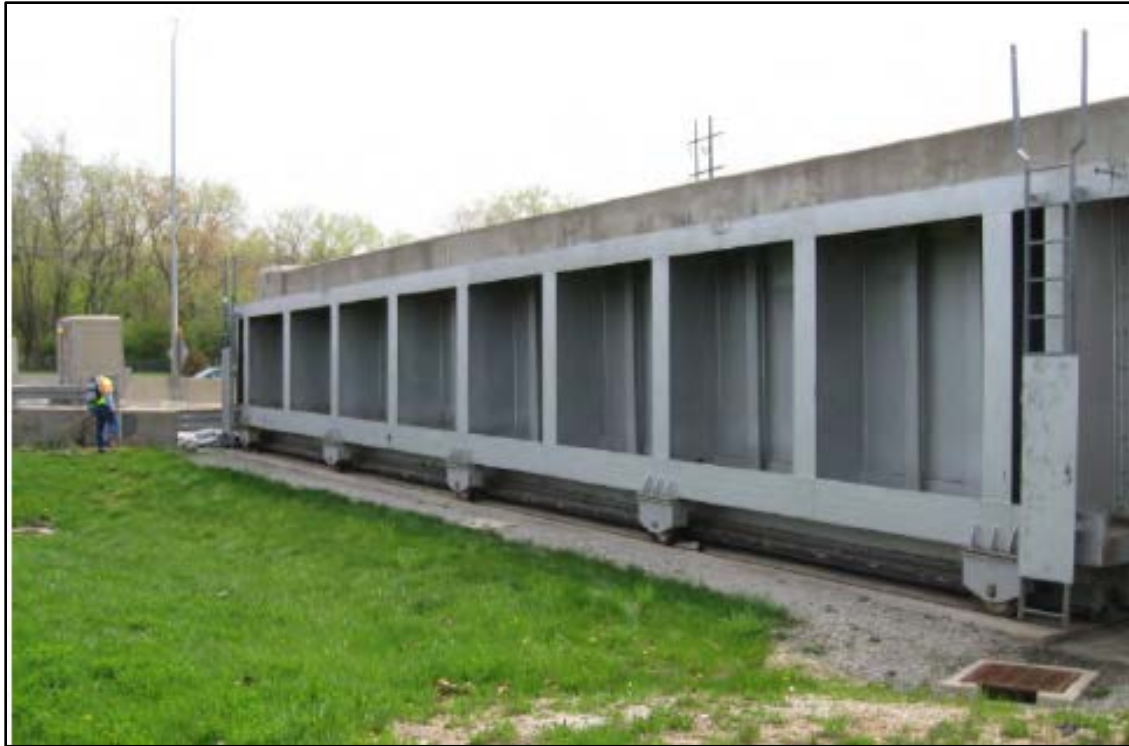
Figure 3-16: Roller Gate (ETL-1110-2-2105)
