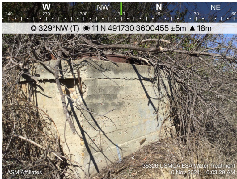
Figure 15. Wire winch wheel and motor with concrete foundation inscribed with the words “Baxter and Peterson,” located near the site's north end.
