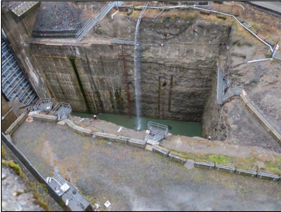
Figure 2. Fish passage facility excavation.
