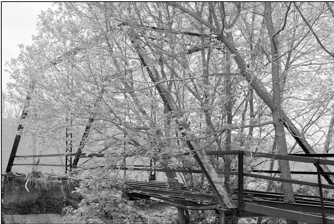
FIGURE 13. ORANGE COUNTY BRIDGE NUMBER 21 PHOTOGRAPH (C. 2005)
