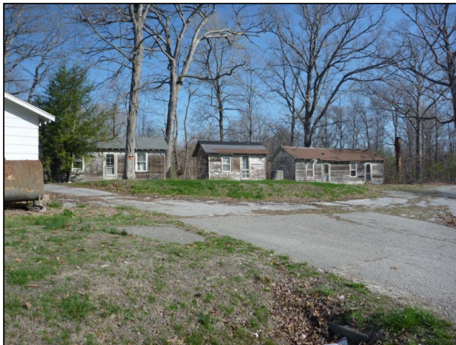
FIGURE 17. SHADY NOOK MOTEL PHOTOGRAPH (C. 2011)
