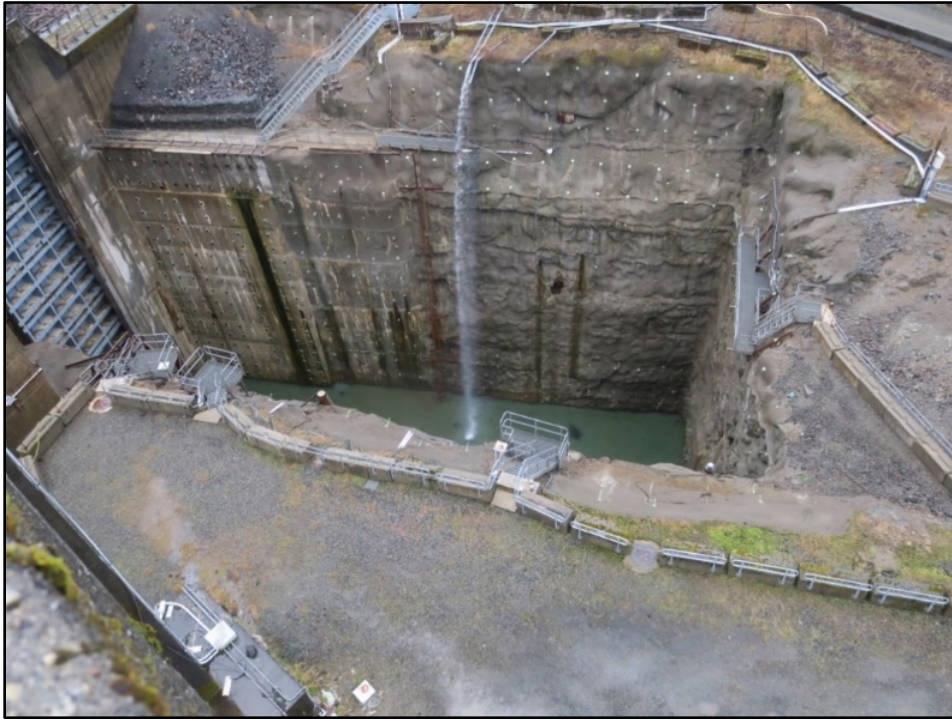
Figure 2. Fish passage facility excavation.
