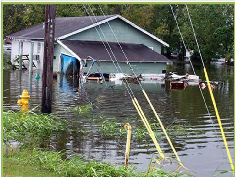
Hurricane Ike flooding in Delcambre, Louisiana 2008.
