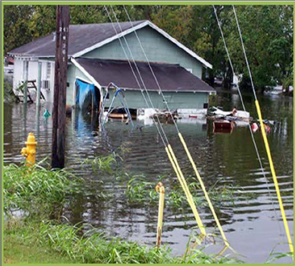
Hurricane Ike flooding in Delcambre, Louisiana.
