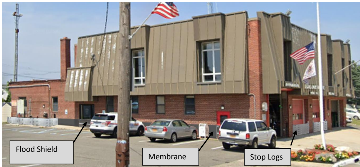
Figure 4: Street View Example of Dry Flood Proofing
