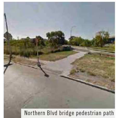
27th Ave overpass entrance
