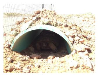
Photo 1: Schedule 80 PVC pipe, 6-feet in length, 3-4 inches of soil/rocks on top to insulate the structure. This is an example of an effective and durable structure.
