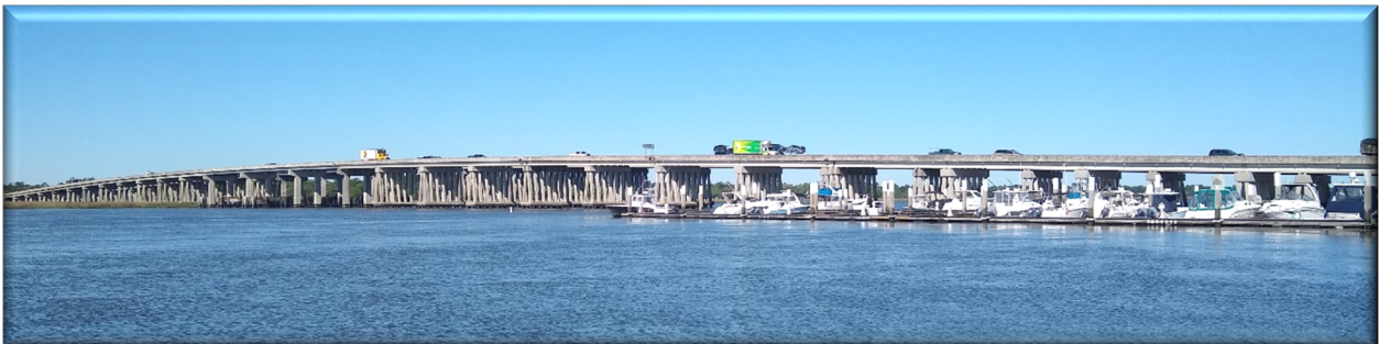
General William C. Westmoreland Bridges over the Ashley River.
