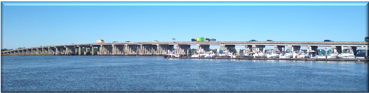
General William C. Westmoreland Bridge over the Ashley River.
