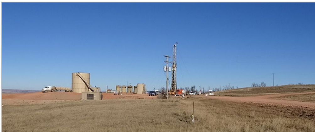
Figure 36. Typical drilling operation and access road with well production operation in the background
