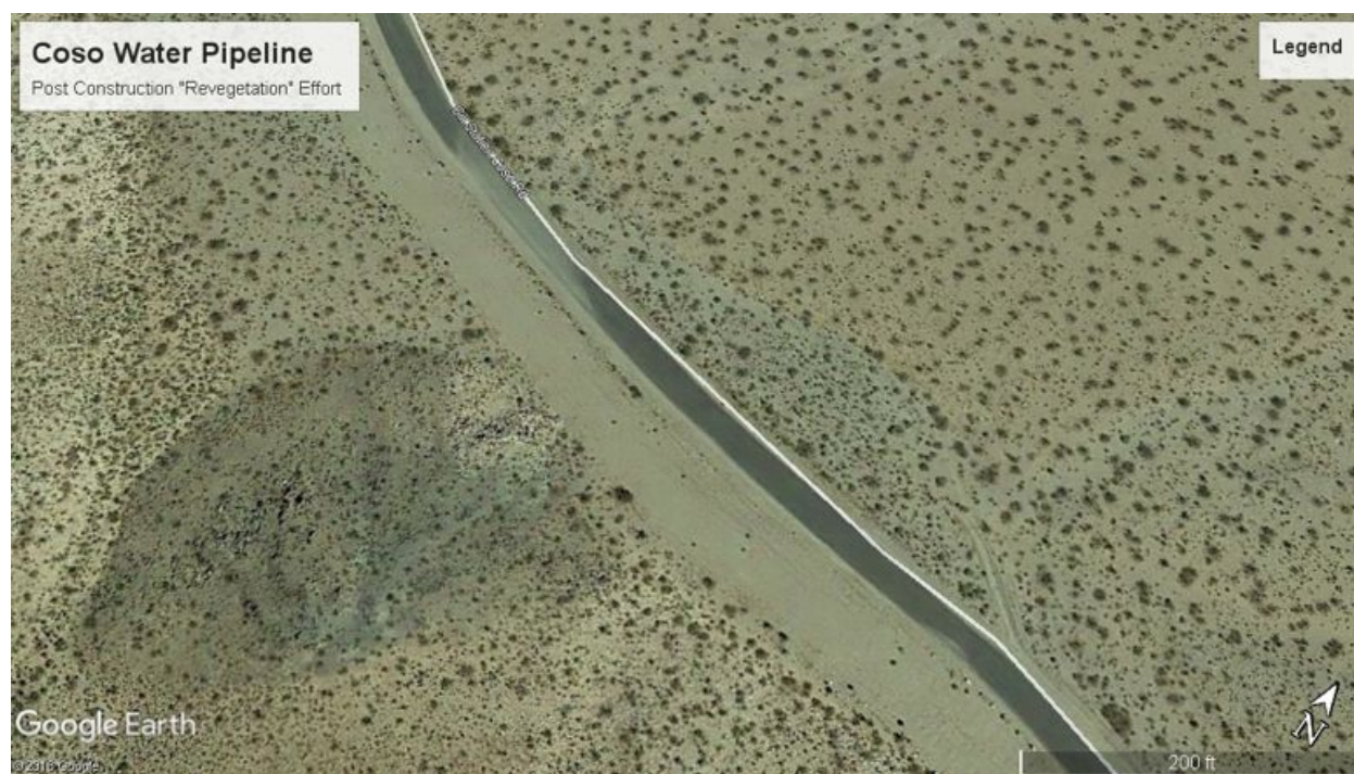
Figure 1. Failed revegetation along the pipeline route of the Hay Ranch Water Extraction and Delivery System by 2017.
