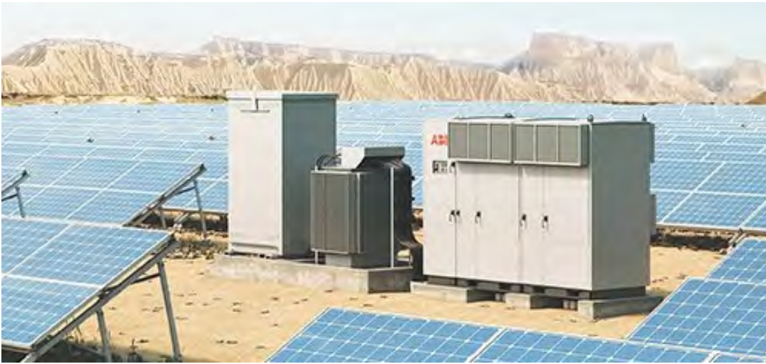
Figure 6. Power conversion station.
