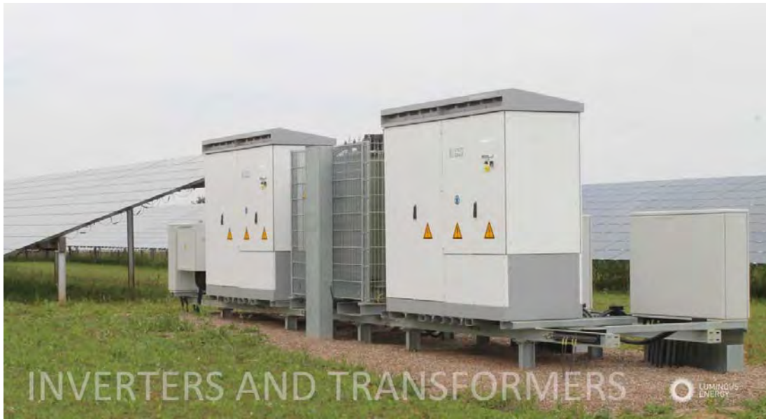
Figure 6 Photographs of a Typical Power Conversion Station/Inverter
