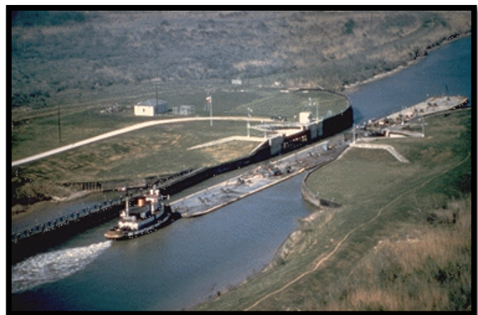
Figure 3-1 – Barged Traffic at CRL
