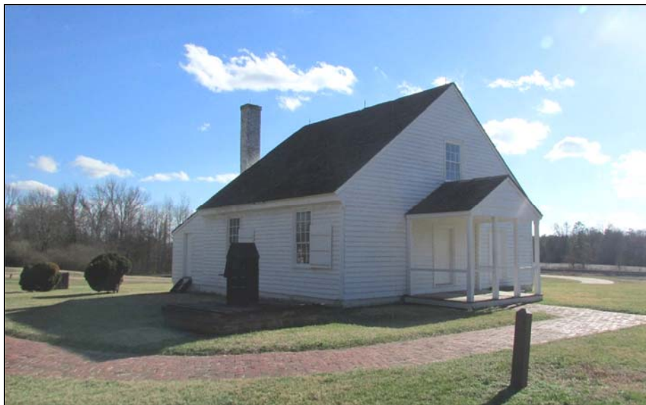
FIGURE 3-40: NORTH OBLIQUE OF SHRINE BUILDING
