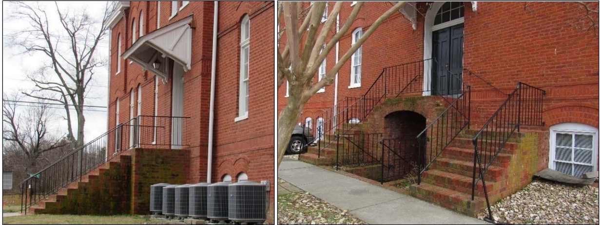
FIGURE 3-214: EAST ENTRANCE, LOOKING SOUTH (LEFT); WEST ENTRANCE, LOOKING NORTHEAST (RIGHT)
