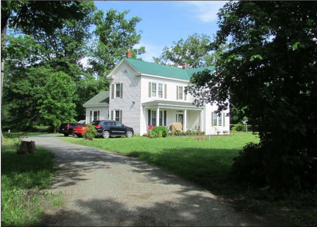
FIGURE 3-160: SOUTHEAST OBLIQUE OF 10536 DOSWELL ROAD (042-0474)
