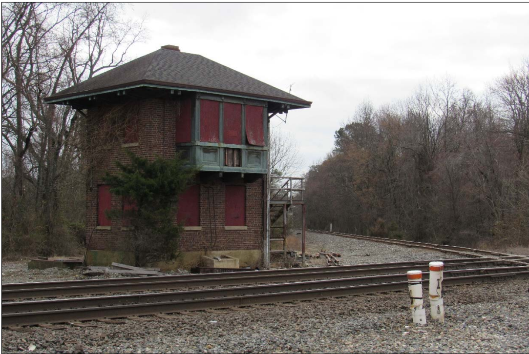
FIGURE 3-204: VIEW OF HN TOWER AND RAILROAD, LOOKING SOUTHEAST
