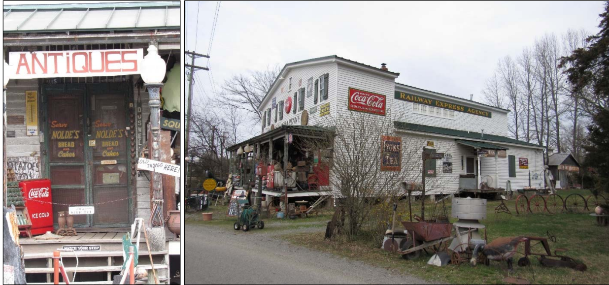
FIGURE 3-169: PRIMARY ENTRANCE DETAIL (LEFT) AND SOUTHEAST OBLIQUE (RIGHT)
