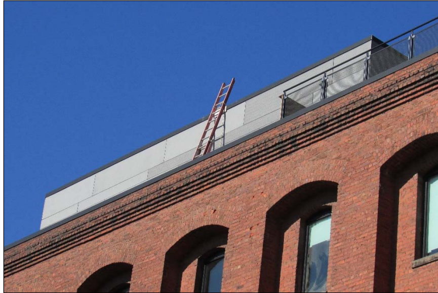
FIGURE 3-269: DETAIL VIEW OF ROOFTOP ADDITION, LOOKING WEST
