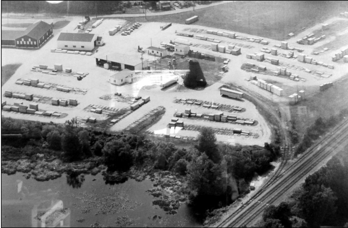
FIGURE 3-105: AERIAL IMAGE OF THE EXCELSIOR OPERATION AT THE DEJARNETTE LUMBER COMPANY TAKEN IN THE 1960S, LOOKING SOUTH (DEJARNETTE LUMBER COMPANY 1960S)
