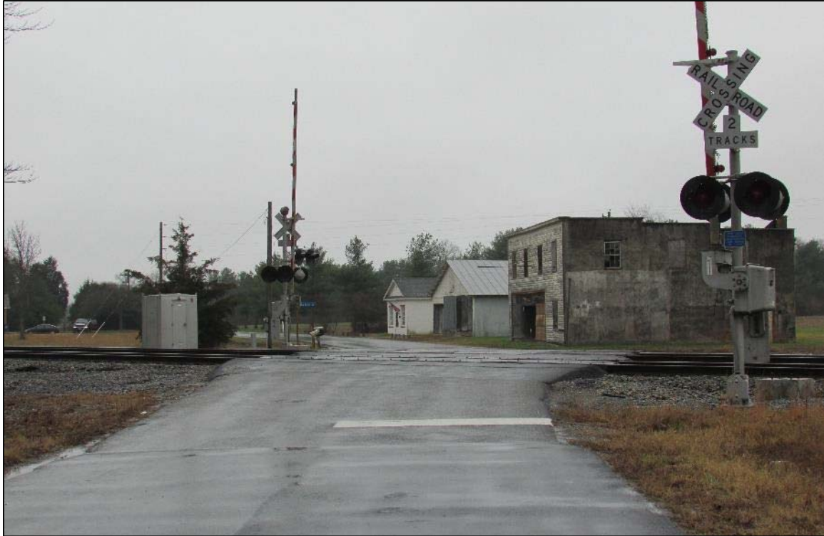
FIGURE 3-57: OVERVIEW OF THE WOODFORD HISTORIC DISTRICT, WHERE WOODFORD ROAD CROSSES THE TRACKS OF THE RF&P RAILROAD, LOOKING SOUTHWEST
