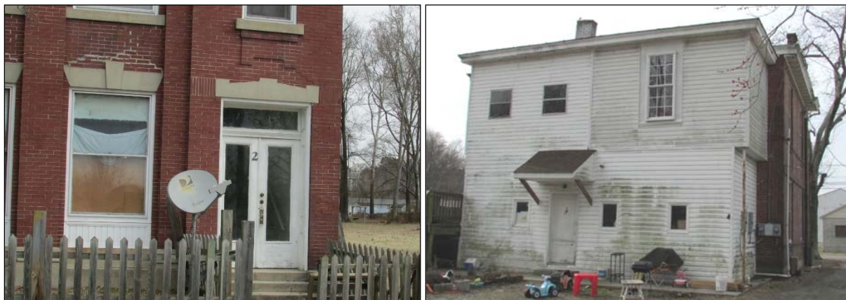
FIGURE 3-134: DETAIL OF FENESTRATION, SOUTHWEST ELEVATION (LEFT); NORTHEAST ADDITION OF THE MILFORD STATE BANK (RIGHT)
