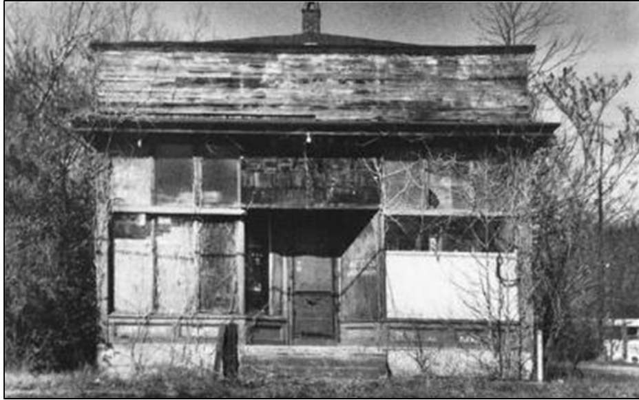
FIGURE 3-118: CIRCA-2011 PHOTOGRAPH OF A COMMERCIAL BUILDING ALONG COLONIAL ROAD (016-0263), NO LONGER EXTANT (FISHER AND SPARENBERG 2011)
