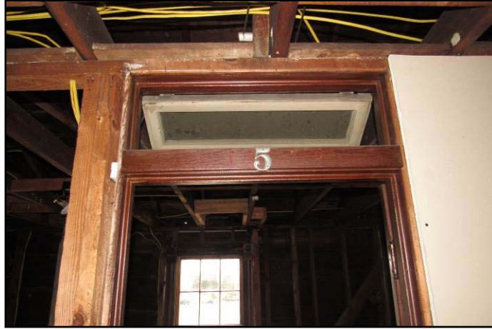
FIGURE 3-192: DETAIL OF ROOM NUMBER, SECOND STORY
