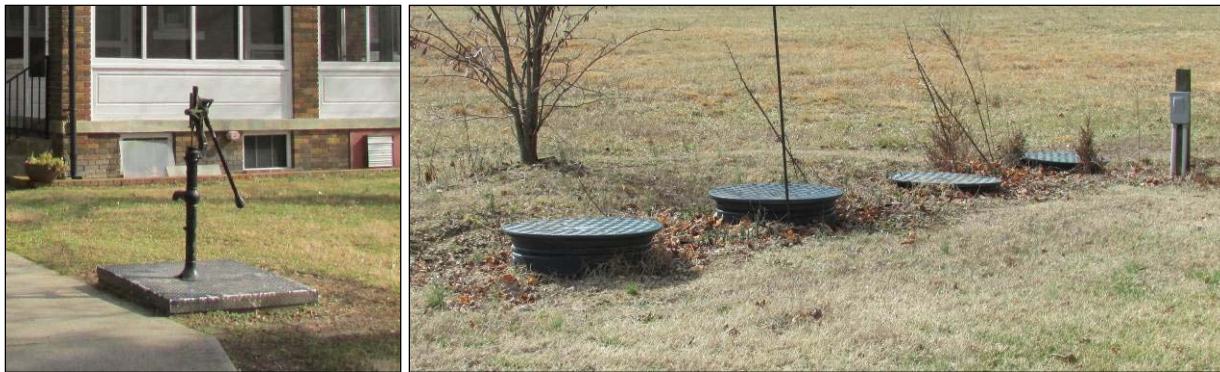
FIGURE 3-91: WELL PUMP, LOOKING EAST (LEFT); FOUR WELLS, LOOKING SOUTHWEST (RIGHT)
