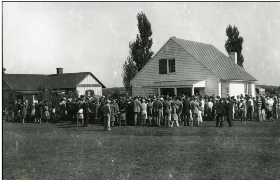
FIGURE 3-37: THIS PHOTOGRAPH, TAKEN IN 1937 ON OPENING DAY, SHOWS THE ENTRY PORCH AS COVERING BOTH DOORS ON THE PRIMARY ELEVATION, AND A SECONDARY STRUCTURE IMMEDIATELY TO THE NORTH (LIBRARY OF VIRGINIA 1937B)
