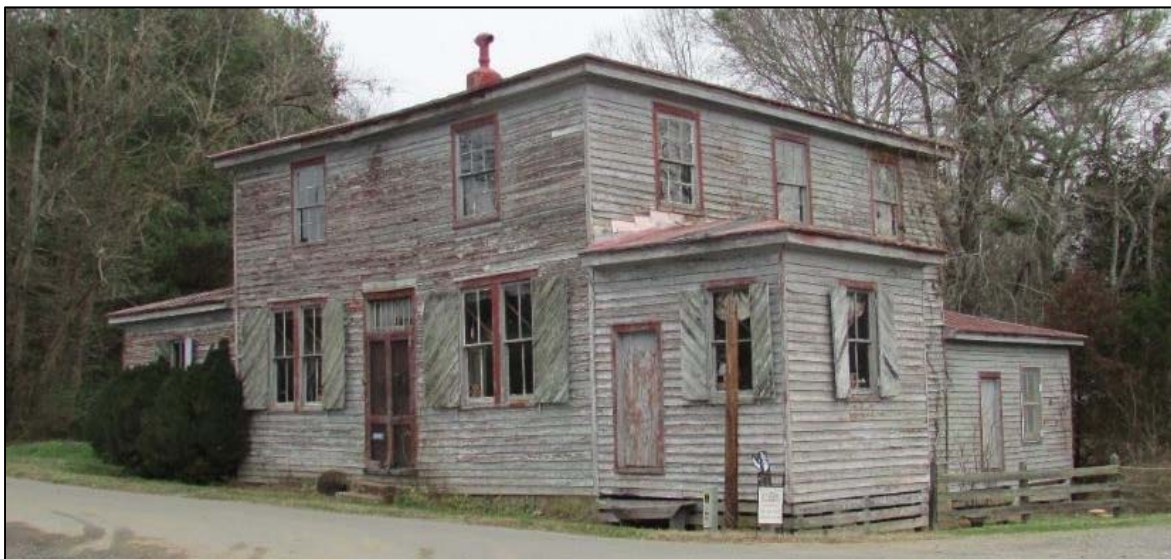
FIGURE 3-139: STORE, SOUTH OBLIQUE
