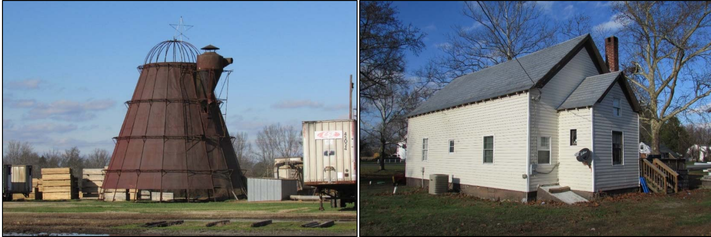
FIGURE 3-122: DEJARNETTE LUMBER COMPANY TEEPEE WASTE BURNER (016-5137), LOOKING NORTH (LEFT); MILFORD PRESBYTERIAN CHURCH (016-0264) NOW CONVERTED TO A RESIDENCE, LOOKING NORTH (RIGHT)
