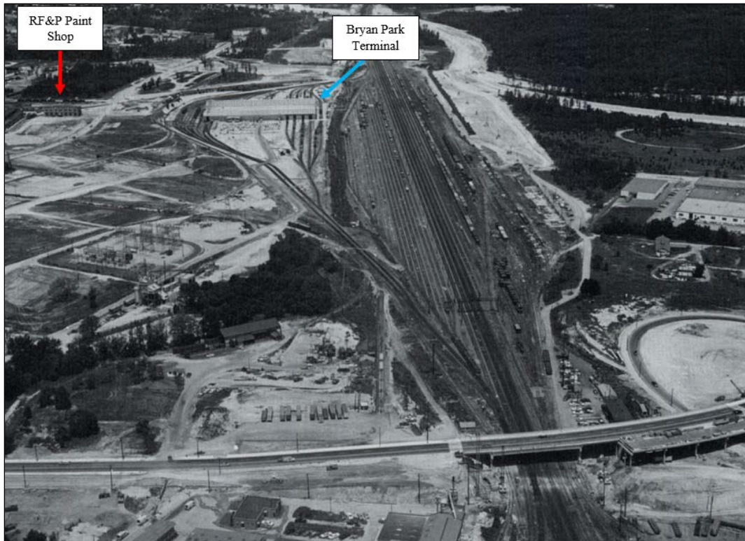
FIGURE 3-221: AERIAL VIEW LOOKING NORTH OF THE ACCA YARD AND BRYAN PARK TERMINAL (DENOTED IN BY BLUE ARROW) TAKEN IN JULY OF 1965 (GRIFFIN 1994:127). RF&P PAINT SHOP DENOTED BY RED ARROW.
