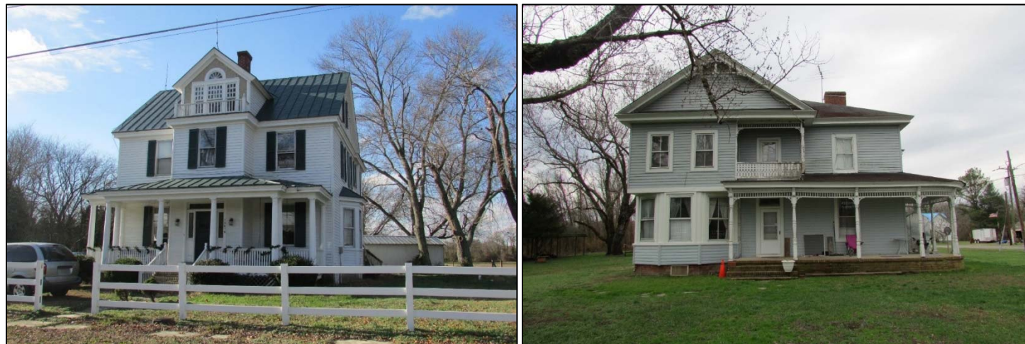
FIGURE 3-125: OLD MILFORD HOTEL (016-0262), NOW A PRIVATE RESIDENCE, LOOKING WEST (LEFT) AND HOUSE AT 15510 NELSON HILL ROAD (016-0267), LOOKING WEST (RIGHT)
