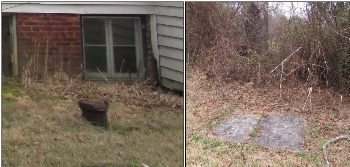
FIGURE 3-194: VIEW OF METAL SUPERSTRUCTURE, LOOKING NORTHWEST (LEFT); VIEW OF STONE SLAB, LOOKING EAST (RIGHT)
