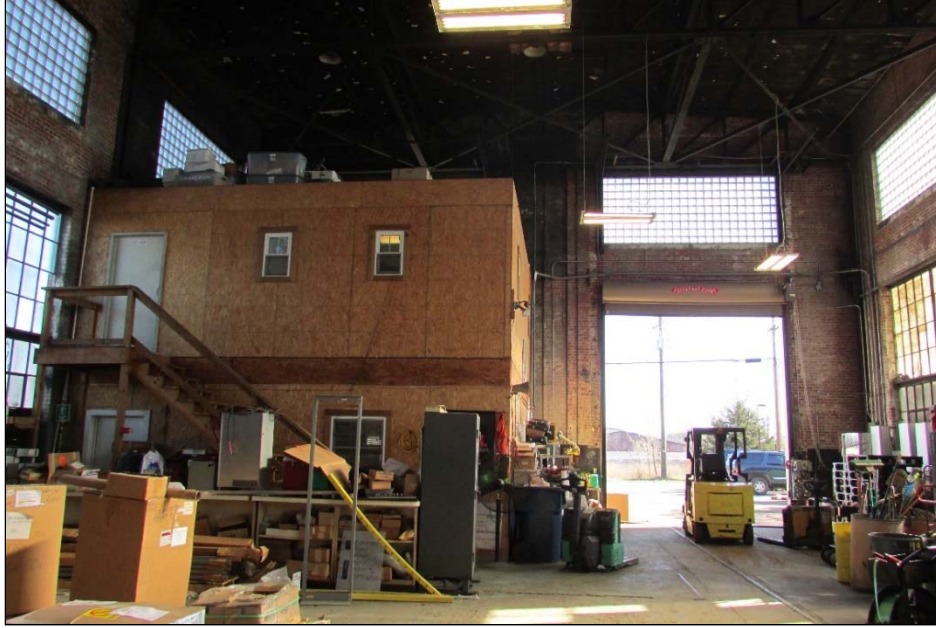
FIGURE 3-230: VIEW OF BUILDOUT AND PRIMARY ENTRANCE, LOOKING NORTHEAST. NOTE DEFUNCT TRACK LINES IN BOTTOM RIGHT OF IMAGE.
