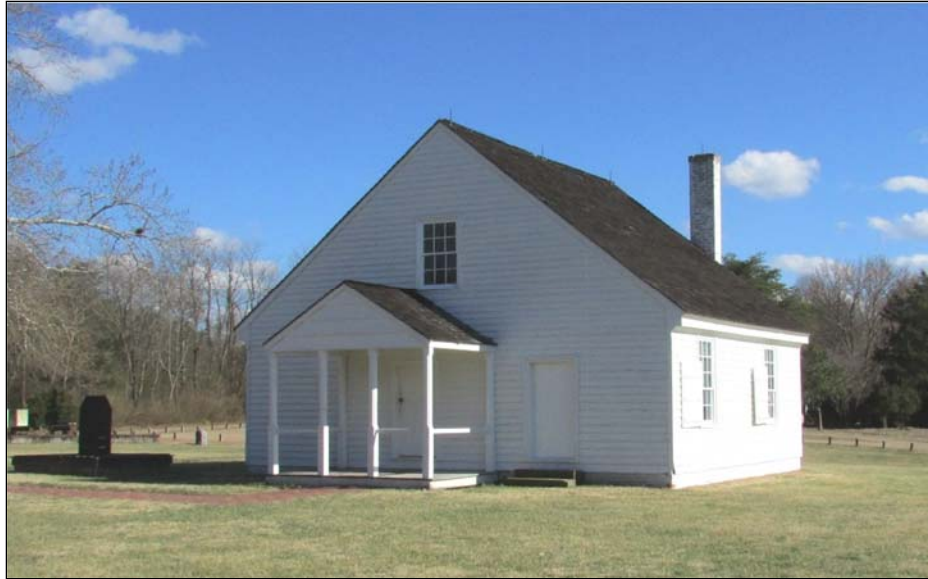
FIGURE 3-39: WEST OBLIQUE OF SHRINE BUILDING
