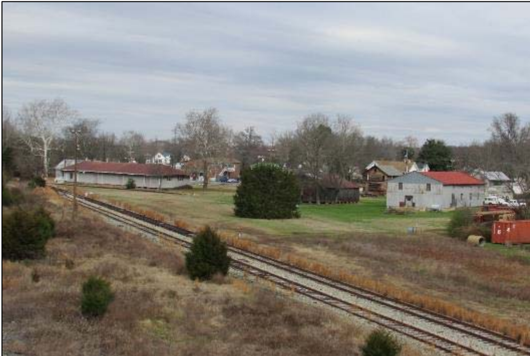
FIGURE 3-121: OVERVIEW OF THE MILFORD HISTORIC DISTRICT WITH MILFORD FREIGHT DEPOT (016-0266) IN BACKGROUND, LOOKING NORTHEAST
