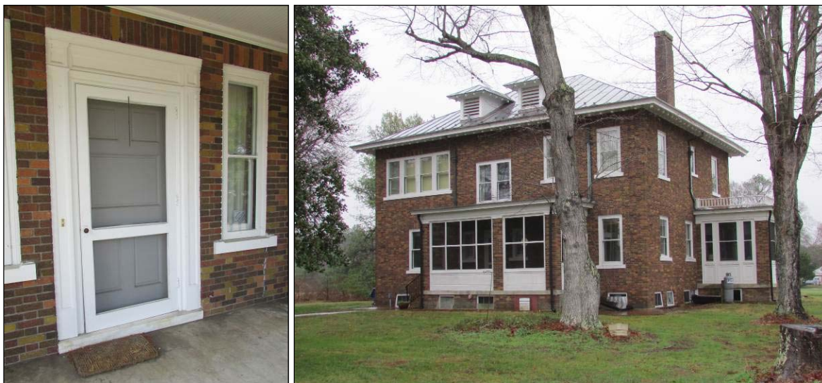
FIGURE 3-89: PRIMARY ENTRANCE, EAST ELEVATION (LEFT); SOUTHWEST OBLIQUE (RIGHT)
