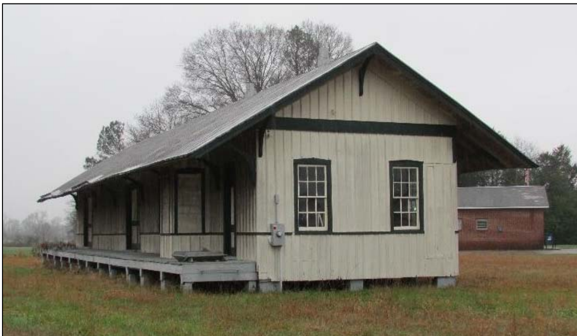
FIGURE 3-58: WOODFORD FREIGHT AND PASSENGER DEPOT (016-0222), LOOKING SOUTH
