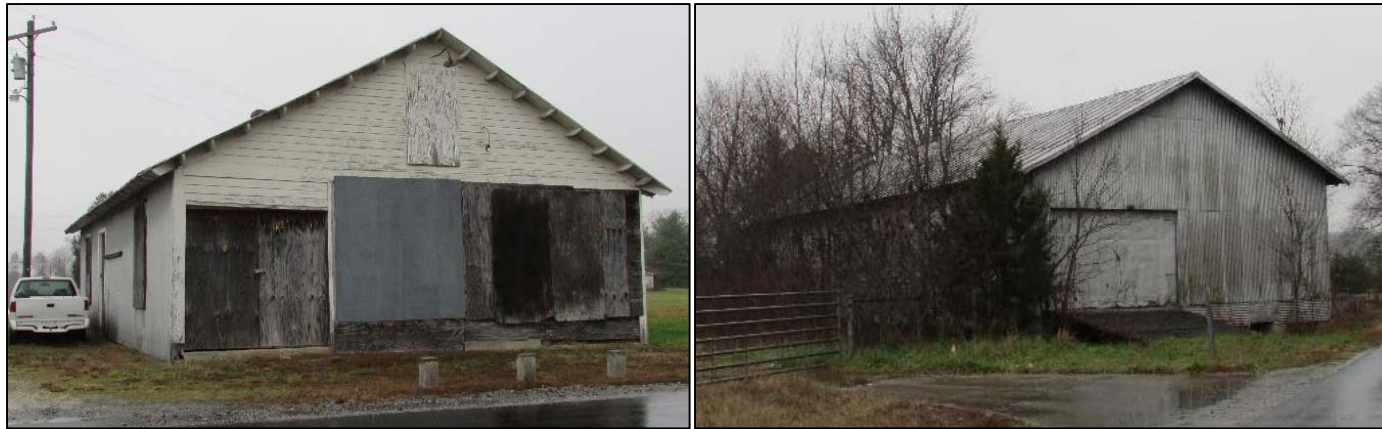
FIGURE 3-61: THE H. WASHINGTON STORE (016-5131), LOOKING NORTHWEST (LEFT); WAREHOUSE (016-5134), LOOKING NORTH (RIGHT)
