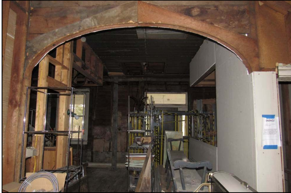
FIGURE 3-188: FIRST STORY HALL, LOOKING EAST
