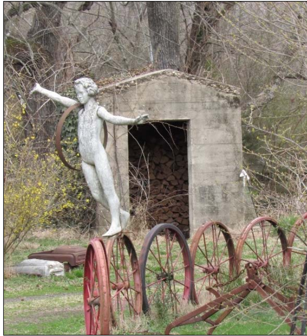
FIGURE 3-171: BATTERY HOUSE, SOUTH ELEVATION
