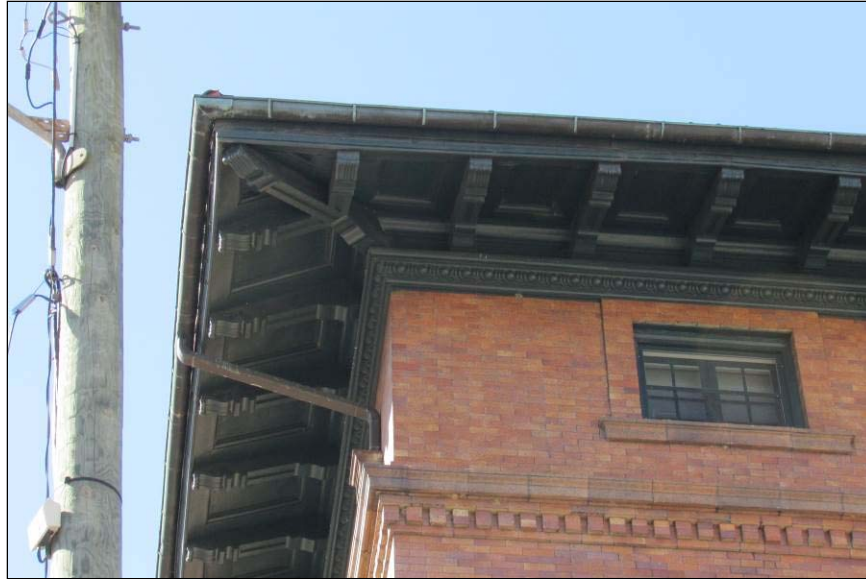
FIGURE 3-251: DETAIL OF EAVE AND CORNICE, WEST CORNER
