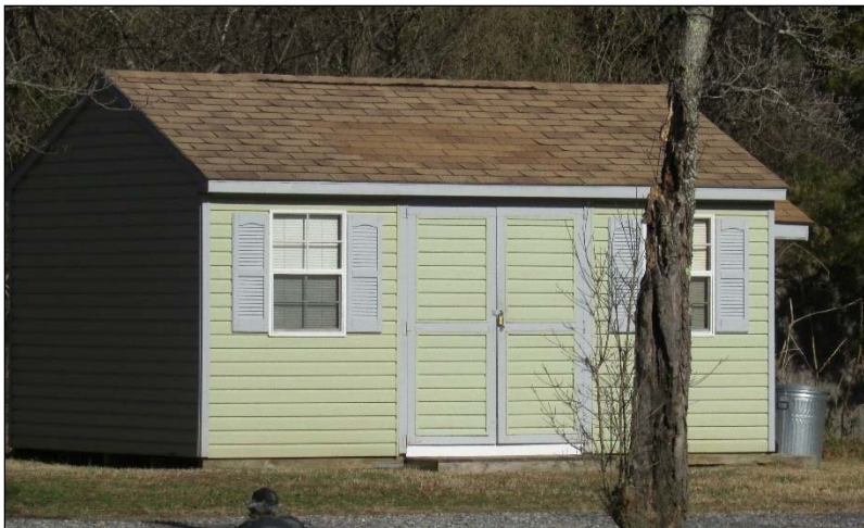
FIGURE 3-48: SHED ASSOCIATED WITH PRIVATE RESIDENCE
