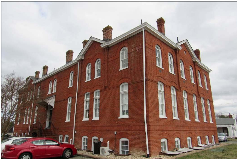
FIGURE 3-212: SOUTHWEST OBLIQUE OF ROBERT STILES BUILDING
