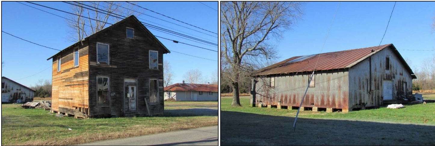
FIGURE 3-124: CLARKS STORE & WAREHOUSE (016-0271), LOOKING WEST (LEFT); CLARKS WAREHOUSE (016-0271), LOOKING WEST (RIGHT)
