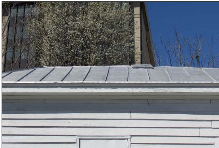
FIGURE 3-237: DETAIL OF FORMER LOCATION OF CHIMNEY, LOOKING NORTHWEST
