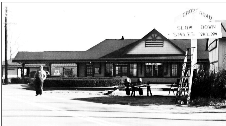
FIGURE 3-76: SEPARATE PASSENGER DEPOT (FRONT) AND FREIGHT DEPOT (REAR) AT MILFORD, CIRCA 1940 (GRAY 1985:98)
