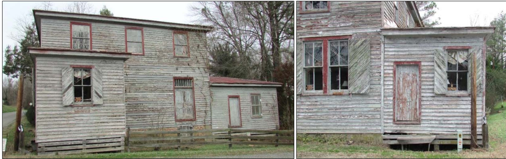
FIGURE 3-140: STORE, SOUTHEAST ELEVATION (LEFT) AND SOUTHWEST ELEVATION AND ADDITION (RIGHT)
