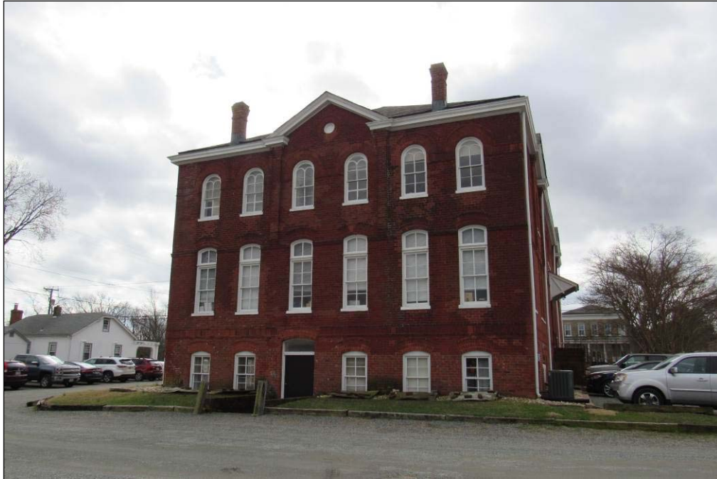
FIGURE 3-213: NORTH ELEVATION OF ROBERT STILES BUILDING
