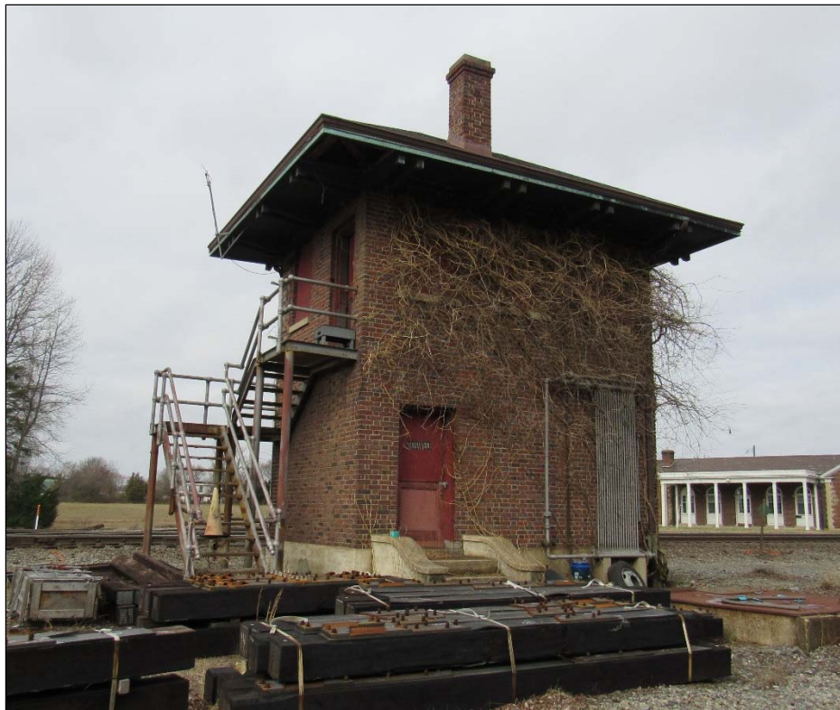
FIGURE 3-205: SOUTHEAST OBLIQUE OF THE HN TOWER
