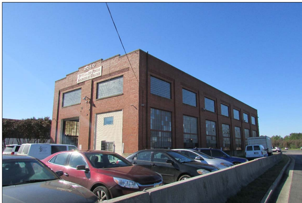
FIGURE 3-226: NORTH OBLIQUE OF THE RF&P PAINT SHOP
