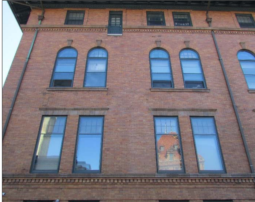
FIGURE 3-253: DETAIL OF FENESTRATION, NORTHWEST ELEVATION
