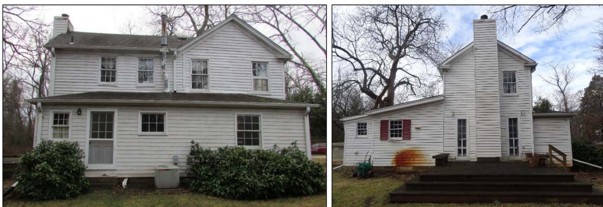
FIGURE 3-28: NORTHWEST ELEVATION (LEFT); NORTHEAST ELEVATION (RIGHT)
