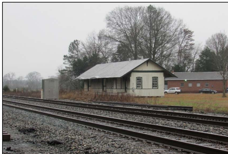
FIGURE 3-80: WOODFORD FREIGHT & PASSENGER DEPOT, VIEW SOUTH FROM RAILROAD CROSSING
