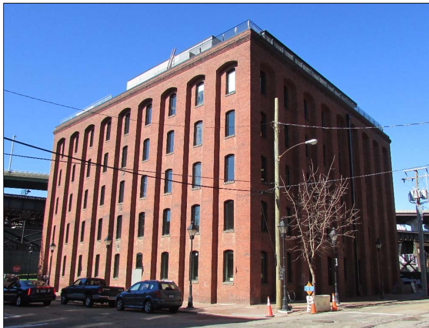
FIGURE 3-267: EAST ELEVATION OF THE PHILIP MORRIS STORAGE WAREHOUSE
