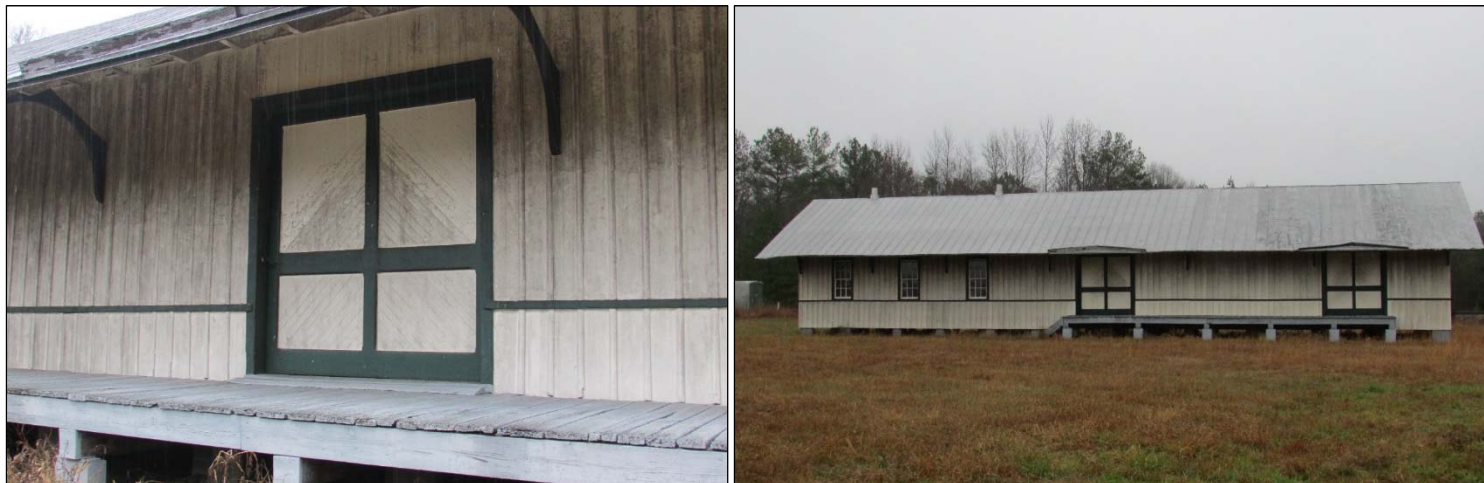
FIGURE 3-82: DETAIL OF SLIDING FREIGHT DOOR ON EAST ELEVATION (LEFT); WEST ELEVATION (RIGHT)
