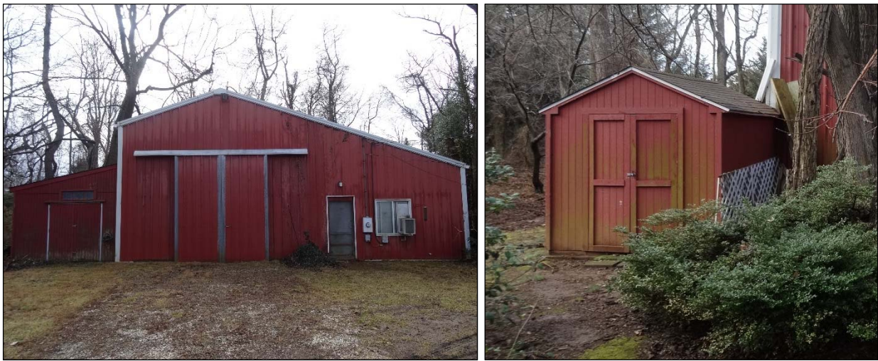
FIGURE 3-29: STUDIO, NORTHEAST ELEVATION (LEFT); SHED, SOUTHEAST ELEVATION (RIGHT)
