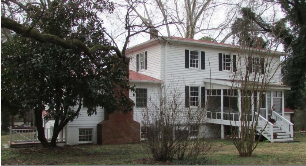
FIGURE 3-148: DWELLING AT 16095 POLECAT LANE, NORTHEAST ELEVATION
