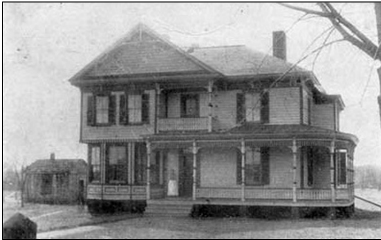
FIGURE 3-113: UNDATED POSTCARD OF THE STILL EXTANT "RESIDENCE OF MRS. J.W. GILL, MILFORD, VA.," LOCATED AT 15510 NELSON HILL ROAD (016-0267) (FISHER 2017)
