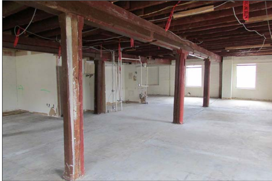
FIGURE 3-12: FIRST STORY INTERIOR, FACING SOUTHEAST
