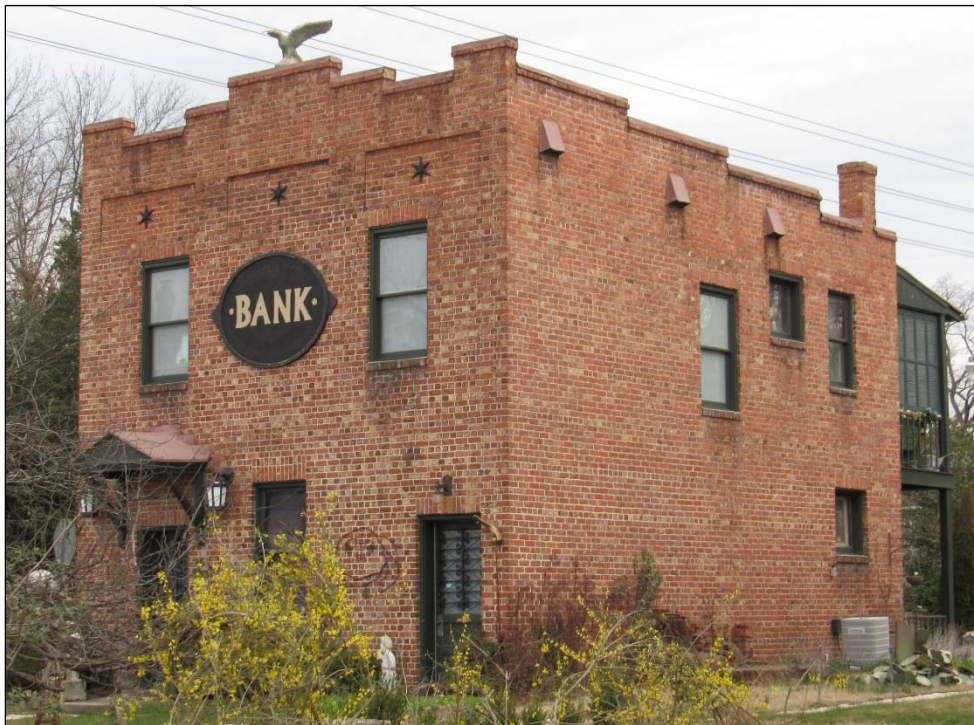
FIGURE 3-177: SOUTHWEST OBLIQUE SHOWING STEPPED PARAPET, PENT ROOF, COMMON AND ENGLISH BRICK BONDS
