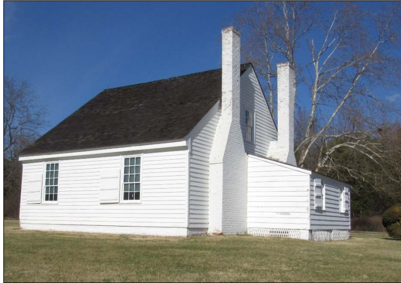
FIGURE 3-41: VIEW OF REAR ADDITION AND EXTERIOR-END BRICK CHIMNEYS, LOOKING NORTH
