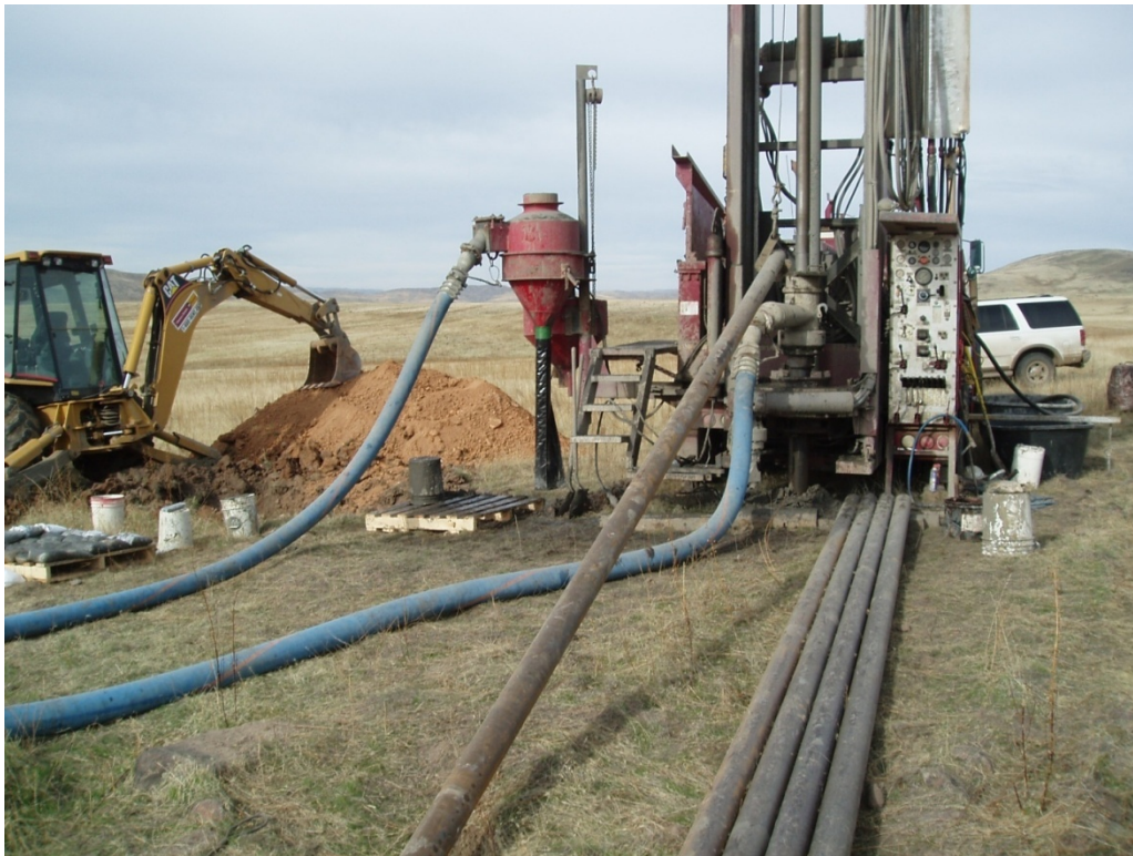
Figure 2. Temperature Gradient Drill Rig at Crane Creek, Fall 2009
