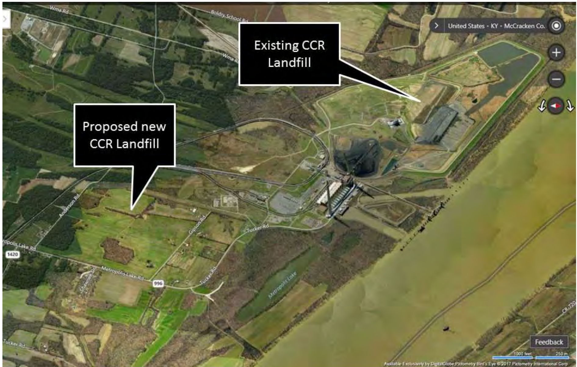
Figure 2. Locations of existing CCR landfill and proposed new CCR landfill. Base image from Bing Birdseye views, view to southeast. Note SHF powerhouse and stacks near center of image.
