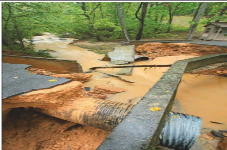
Figure 3-7. Washed Out Road Crossing – Atlanta, GA
