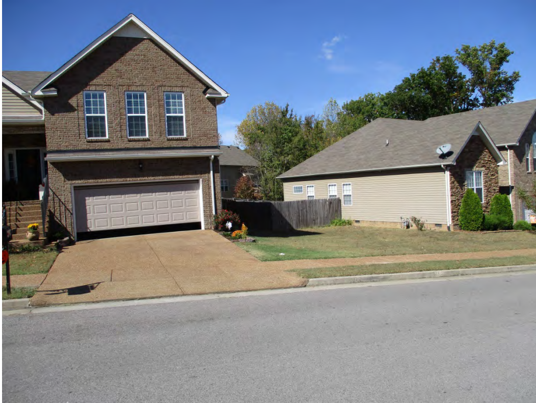
Figure 19. Hidden Creek Subdivision, Photo Point 29
