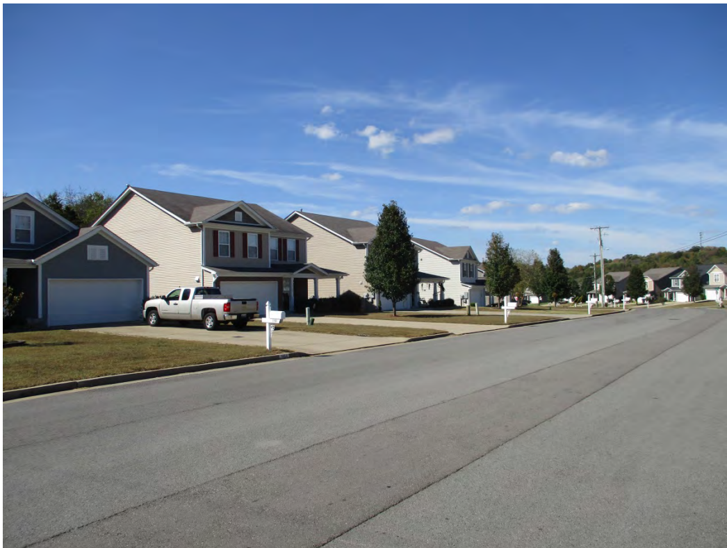
Figure 16. Hidden Creek Subdivision, Photo Point 26
