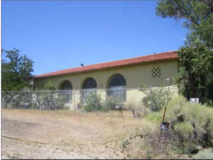
East elevation main Bell Switching Station building, view from SR-138 towards the southwest
