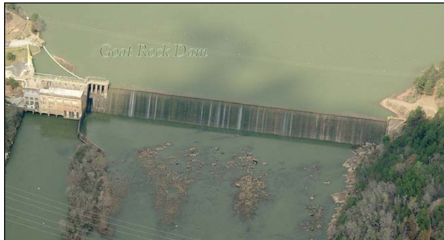
Figure 4-13. Goat Rock Dam (Photograph courtesy of GPC)
