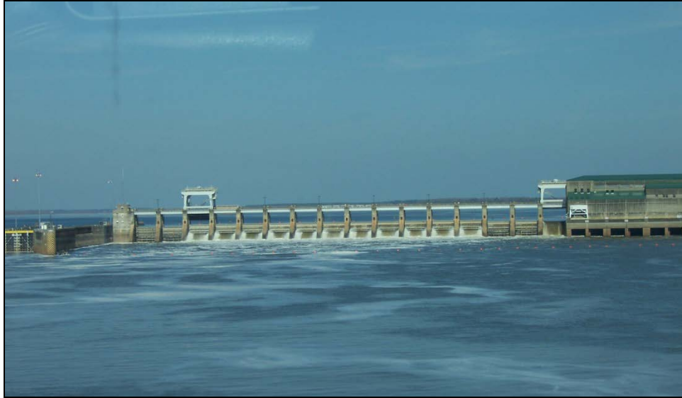
Figure 4-6. Jim Woodruff Lock and Dam
