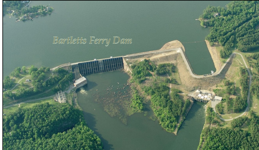
Figure 4-12. Bartletts Ferry Dam (Photograph courtesy of GPC)
