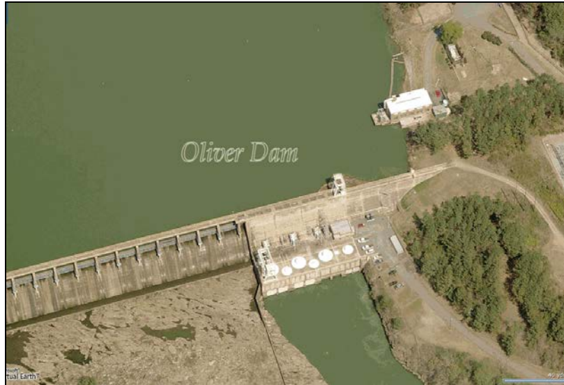
Figure 4-14. Oliver Dam (Photograph courtesy of GPC)
