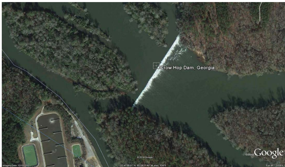
Figure 4-11. Crow Hop Dam (Photograph courtesy of Google Earth)
