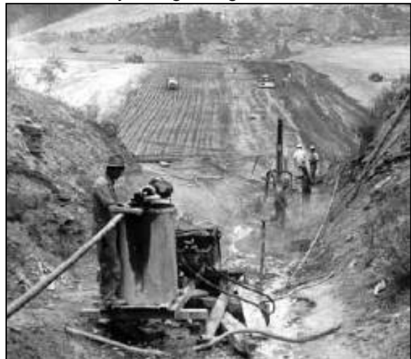
Figure 3-1. Foundation work at Buford Dam (Circa 1950-51)
