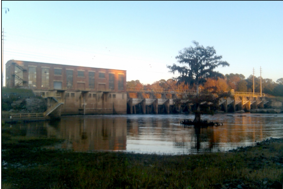
Figure 4-19. Flint River Dam
