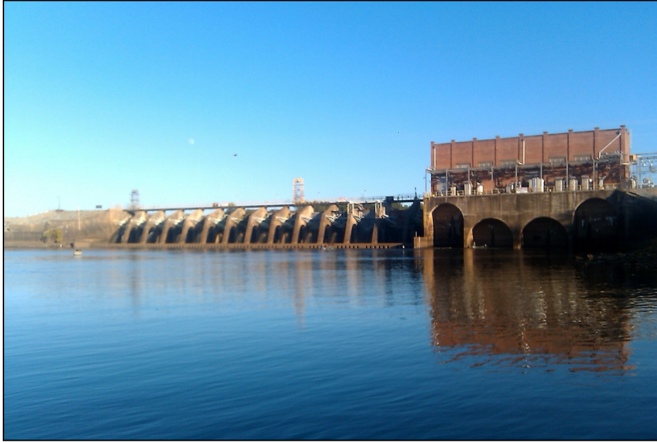
Figure 4-18. Crisp County Dam
