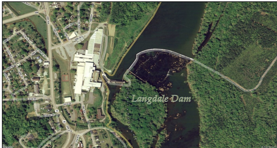
Figure 4-9. Langdale Dam (Photograph courtesy of Google Earth)
