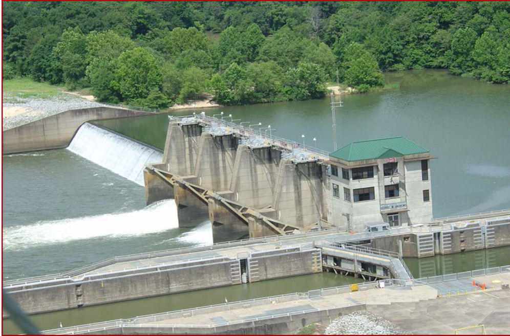
Figure 4-5. George W. Andrews Lock and Dam
