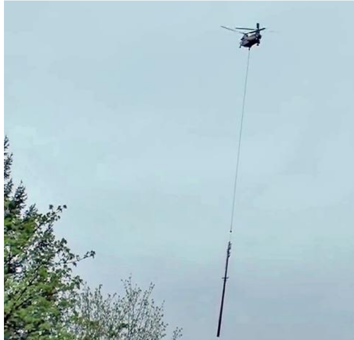
Chinook helicopter transports a replacement structure to a remote portion of transmission line. Photo: BPA
