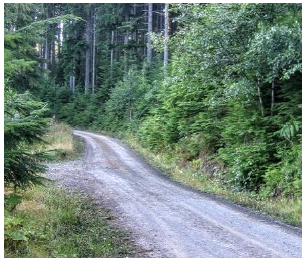
Standard best management practices to minimize erosion include placing crushed surface rock on roads. Photo: DNR
