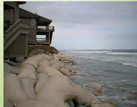
Sandbags protecting a home along the northern portion of Figure Eight Island, March 18, 2008
