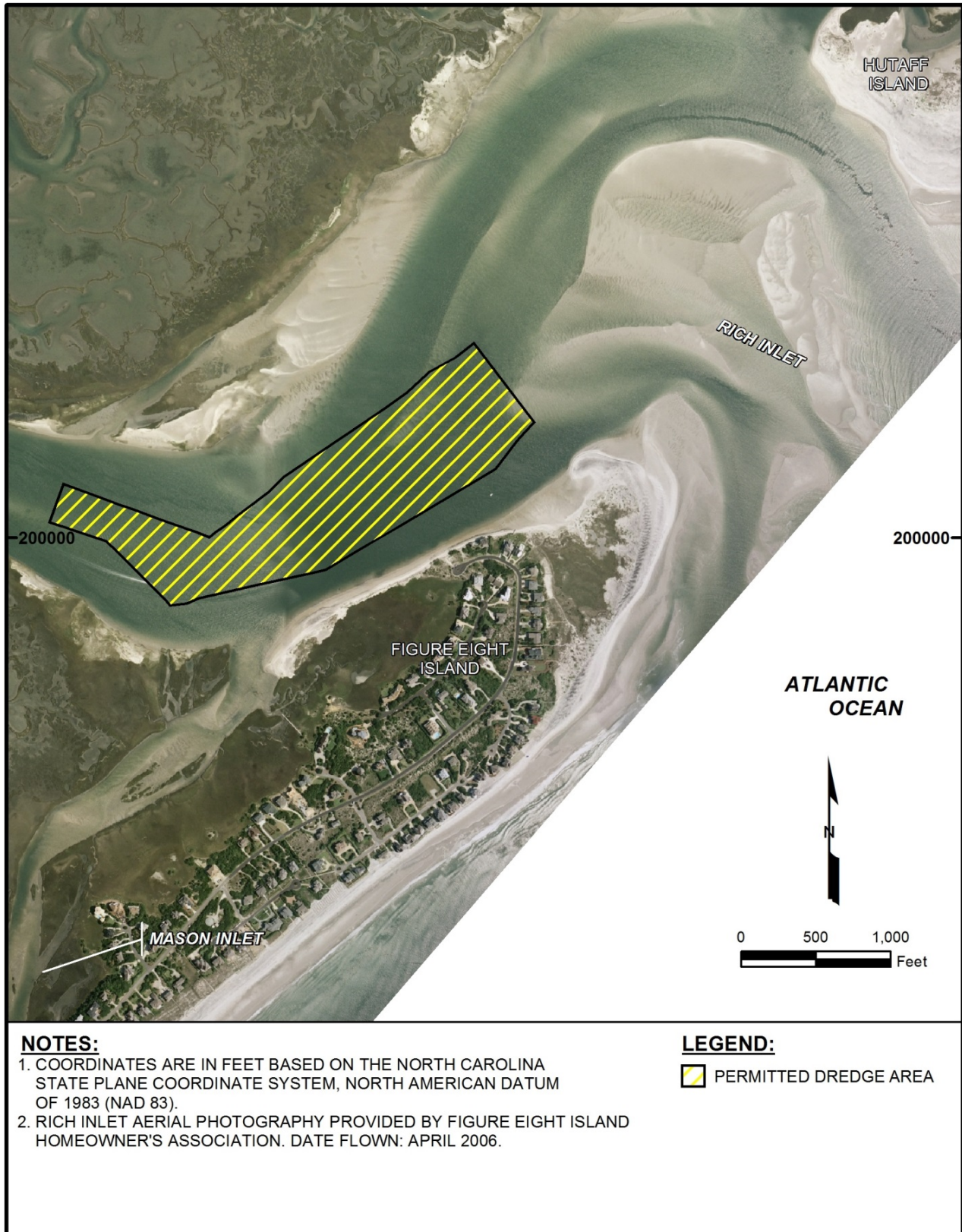
Figure 3.1. Previously permitted dredge area in Nixon Channel.
