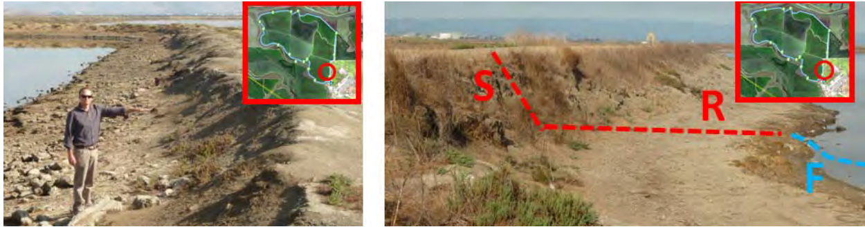
Figure 10 - runout of flow material just beyond the dike toe
