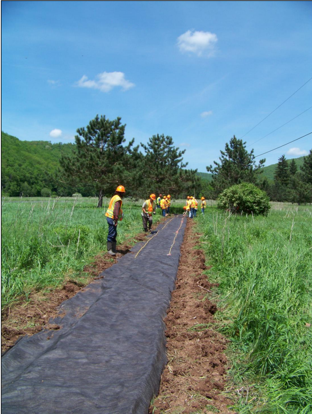
Installation looking north.
