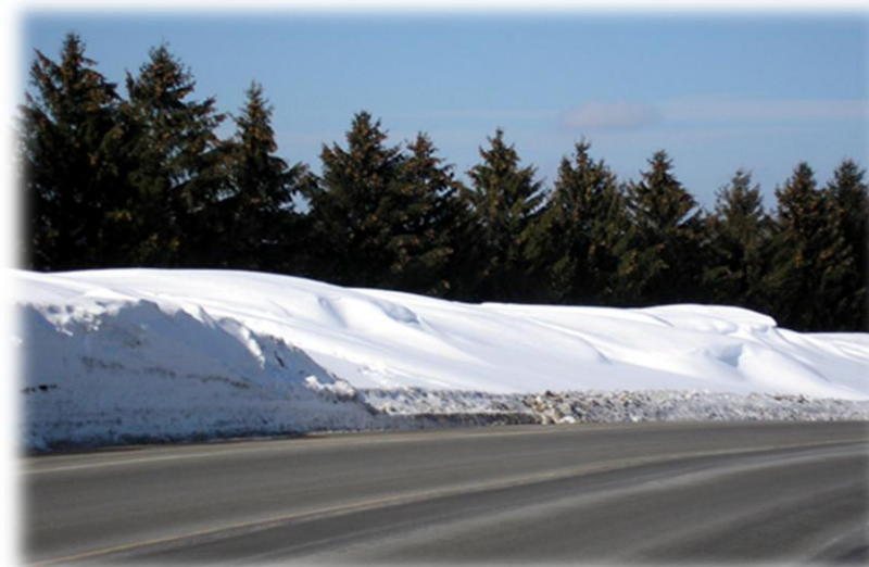
Spruce living snow fence on Rt. 167, Manheim, Herkimer County, NY.
