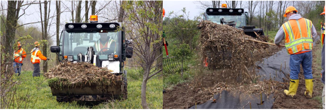
Left picture: Equipment bringing mulch to snow fence from roadside.
