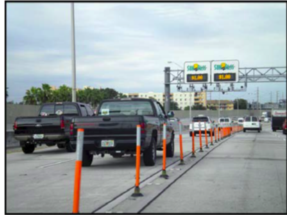
Pylon separation on the I-95 Express in Miami
