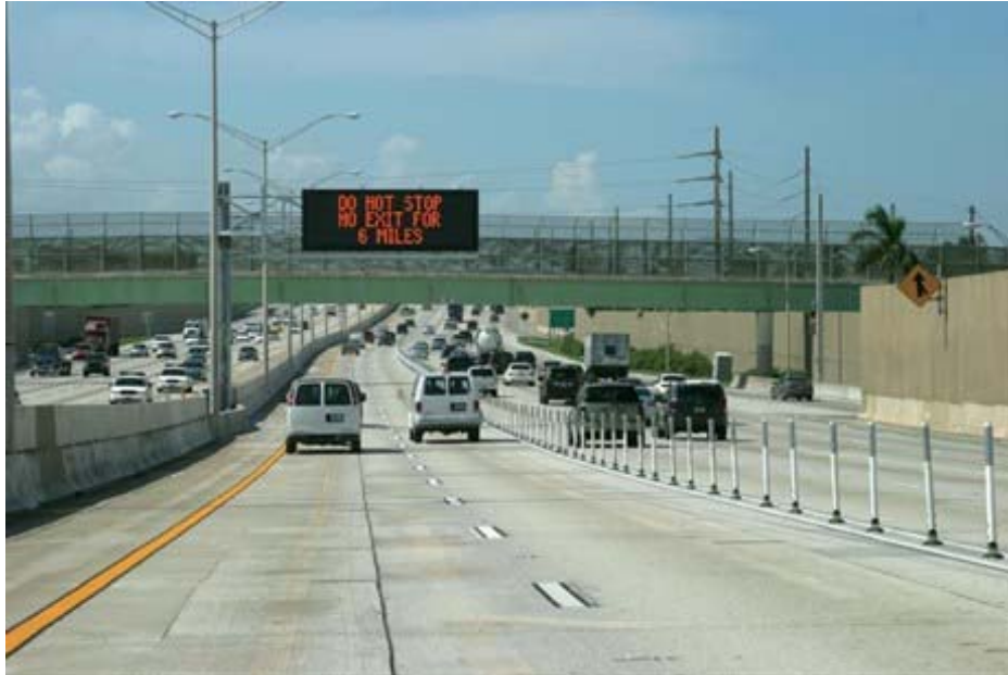
FIGURE 3.19 Buffer Separation on 95 Express, Florida 9
