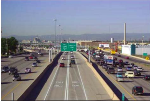
Concrete barrier separation on I-25 Express in Denver
