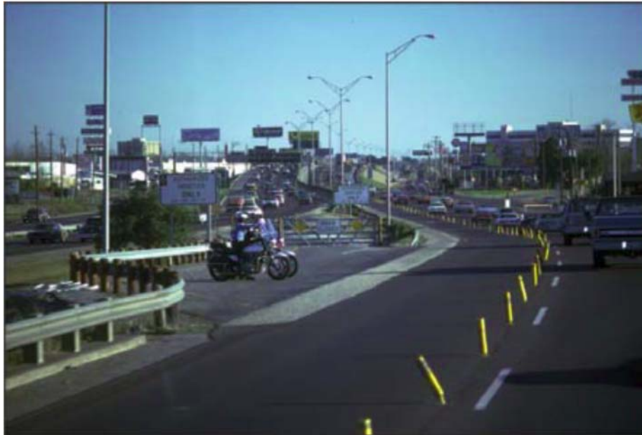
FIGURE 2.10 Enforcement Area on I-45 in Houston
