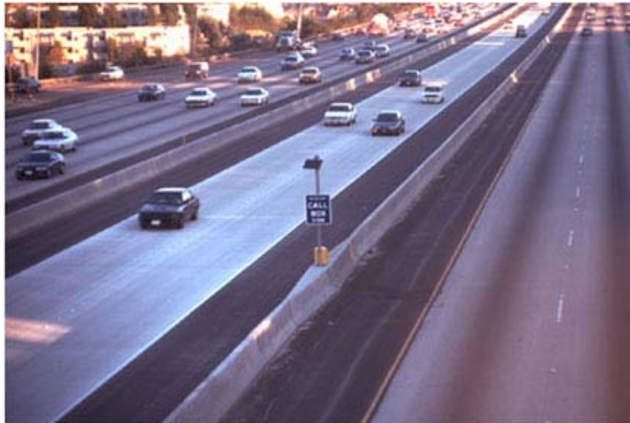
FIGURE 3.20 Concrete Barriers on I-15 Express Lanes, San Diego, California 10
