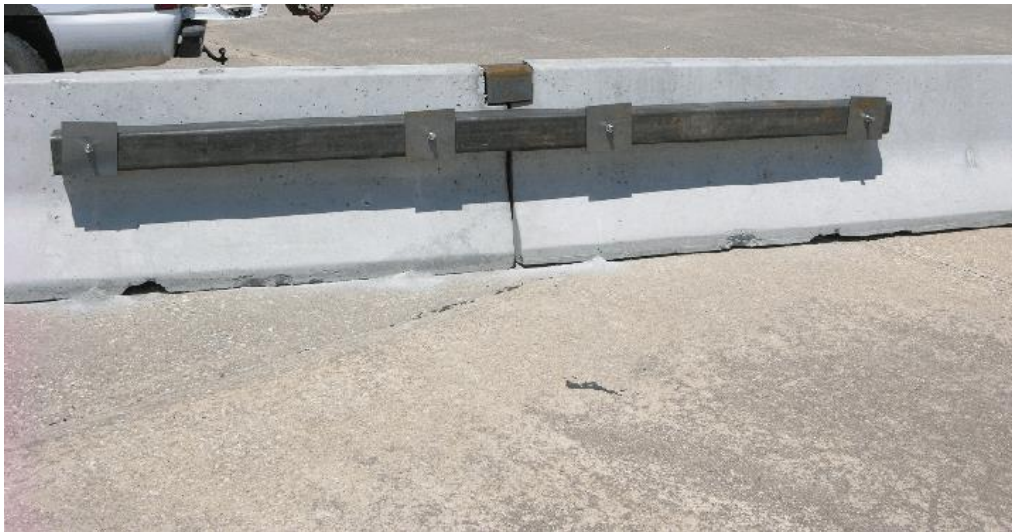
Figure 25. NYSDOT Box-Beam Stiffener System [29]
