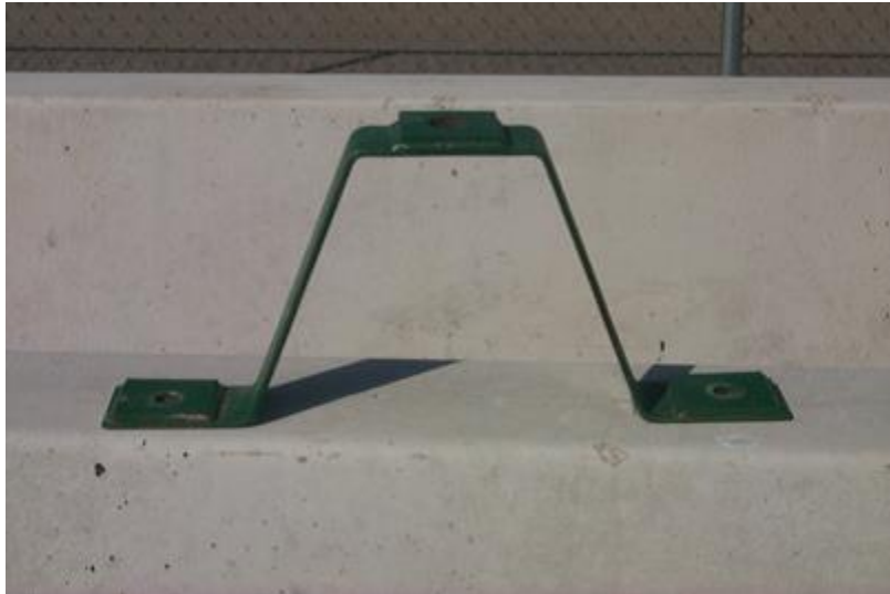
Figure 7. Steel Tie-Down Strap [12]
