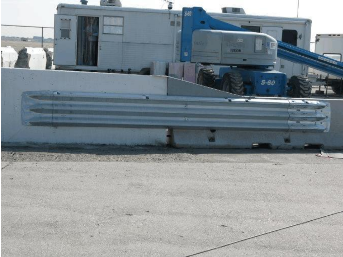
Figure 11. Transition from PCB to Permanent Concrete Barrier [2]
