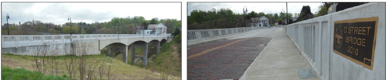
Figure 7. D Street Bridge in Lynchburg
