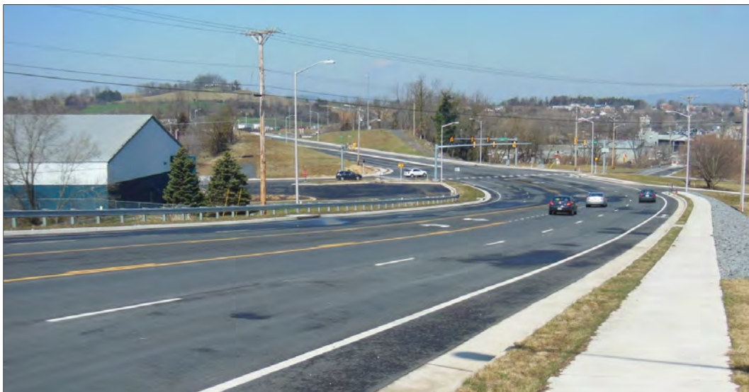
Figure 5. Stone Spring Road in Harrisonburg
