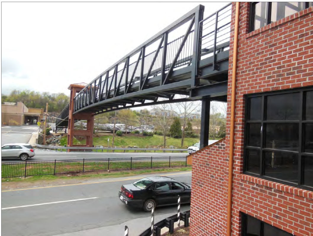
Figure 8. Pedestrian Bridge Over Wards Road in Lynchburg
