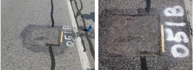
Figure 6.5 Pictures for a Spray Injection Patch after 0, 29, 161, And 188 Days Of Installation
