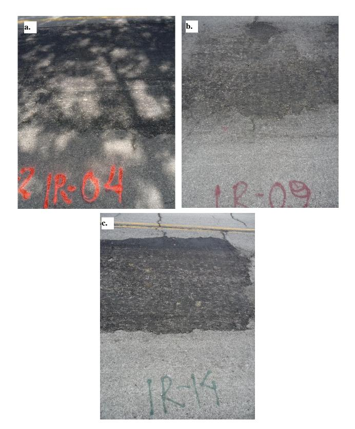
Figure 6.11 Infrared Patches installed on SR 167 after 30 Days of Installation
