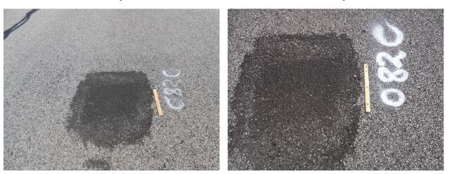
Figure 6.4 Pictures for Infrared Patch after 0, 29, 161, And 188 Days Of Installation
