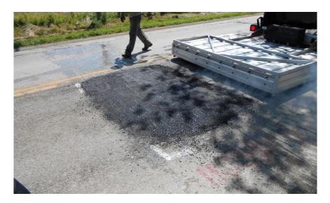
Figure 5.11 Patches Installed Using Infrared Method 1 at SR 168
