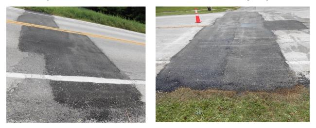
Figure 5.17 Infrared Patches installed at Ohio State Route 18
