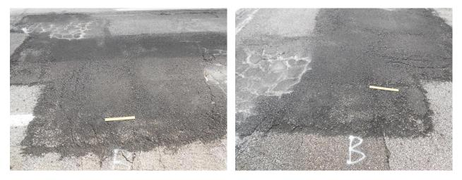
Figure 6.10 Infrared Patches on US 422 after 70 Days of Installation
