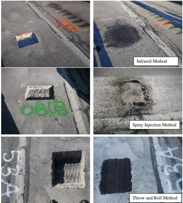
Figure 5.3 Pictures of Potholes Before And After Patch At I-480
