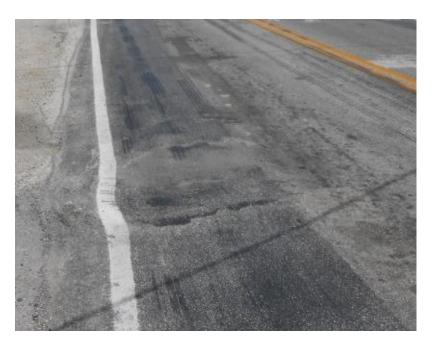
Figure 5.18 Distressed Pavement Area That Was Patched at Ohio SR 635
