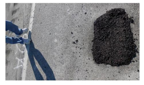
Figure 6.7 Right-After-Construction View Of A Throw And Roll Patch That Performed Well
