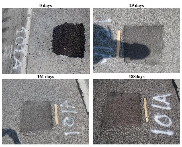
Figure 6.6 Pictures for a Throw-and Roll Patch after 0, 29, 161, And 188 Days Of Installation
