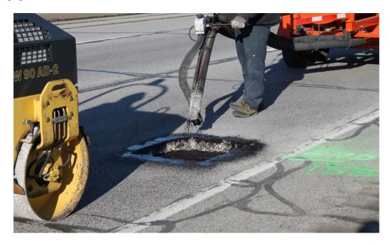
Figure 5.6 A Picture Taken During Patching A Pothole At I-480 Using Spray Injection Method
