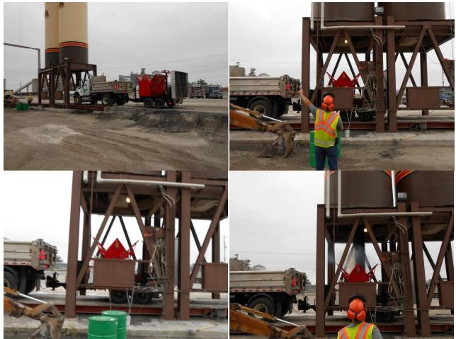
Figure 5.14: Pictures Of Loading The Infrared Reclaimer With Asphalt Materials At The Plant
