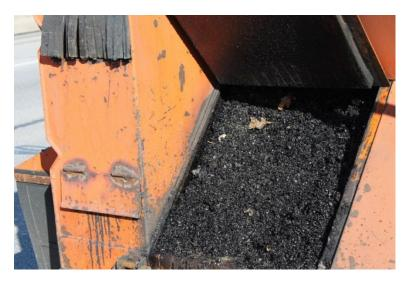
Figure 5.5 Throw-And-Roll Cold Mix Patching Material At I-480
