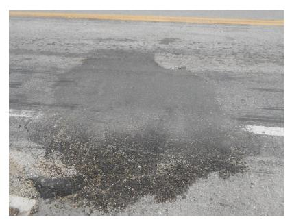
Figure 5.19 Patch Installed Using Infrared at Ohio SR 635
