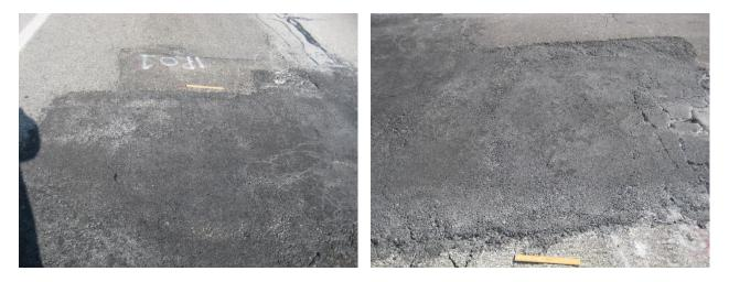
Figure 6.9 Infrared Patches on US 422 after 37 Days of Installation
