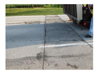
Figure 5.16 One of the Trenches at Ohio State Route 18 Before Repairing It
