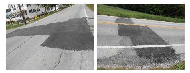
Figure 6.12 Infrared Patches installed on SR 18 after 30 Days of Installation
