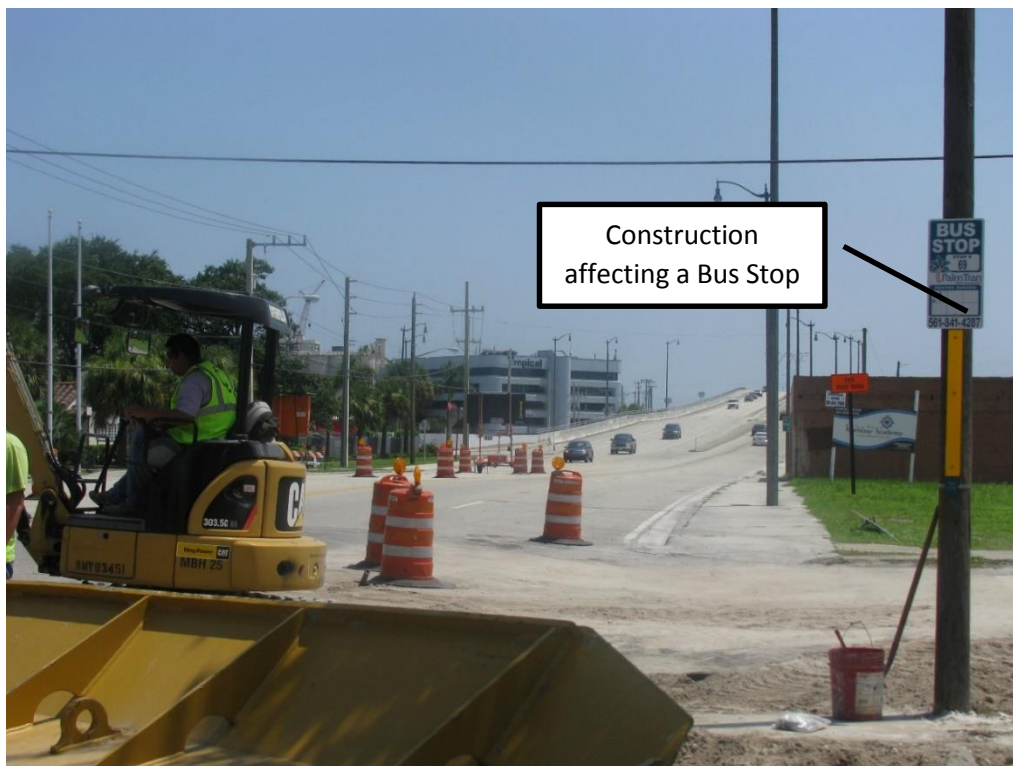
Figure 7-1: Construction Affecting a Bus Stop (Palm Beach)
