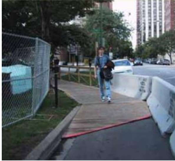
Figure 5-14: Work Zone Accessibility
