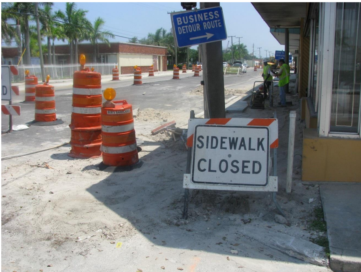
Figure 5-15: Sidewalk Closed Due to Construction
