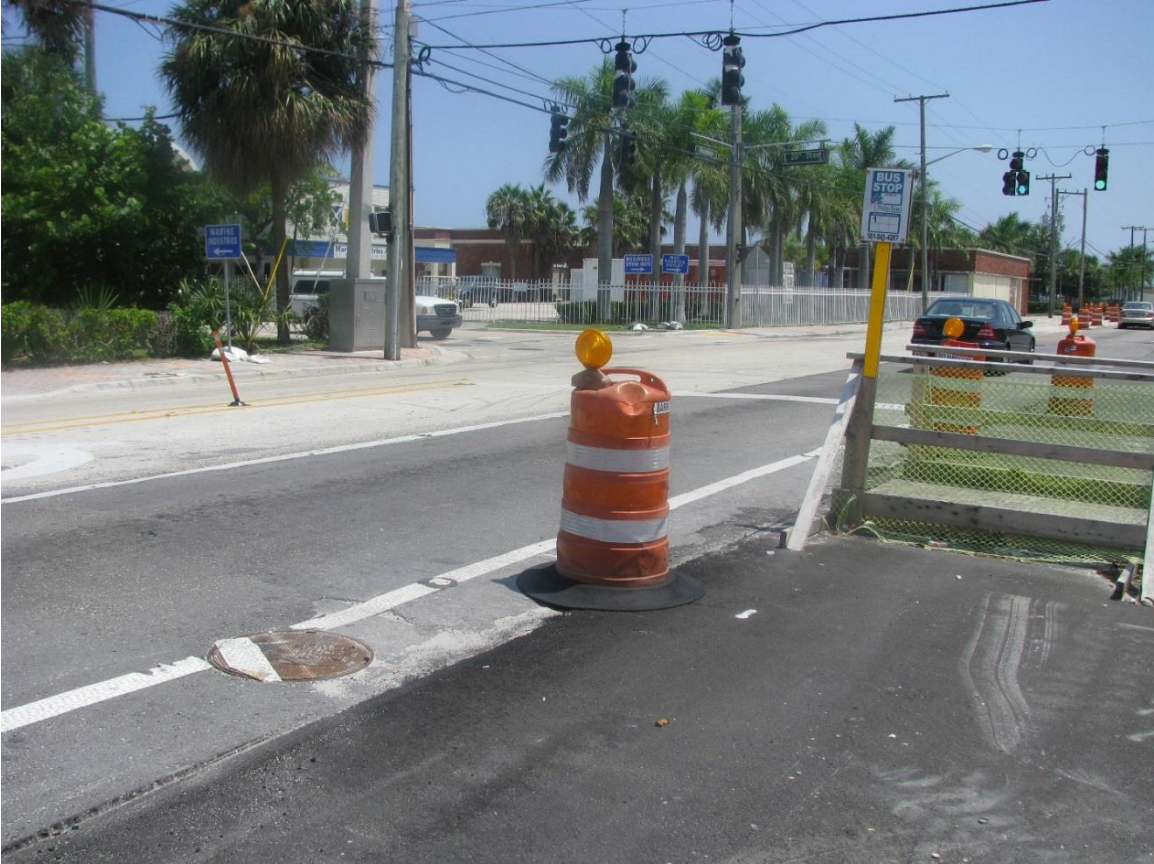
Figure 7-5: Bus Stop at a Construction Zone
