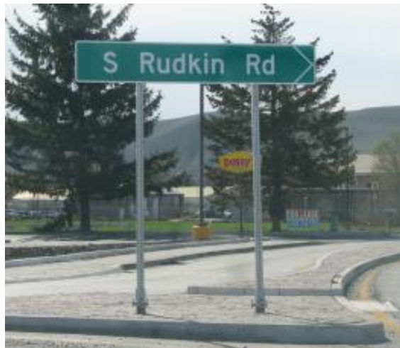
FIGURE 5.6 A Removable Sign on Roundabout Splitter Island
