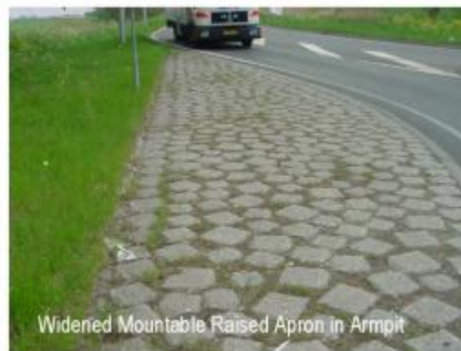
FIGURE 5.18 Cobblestone External Truck Apron in the Netherlands
