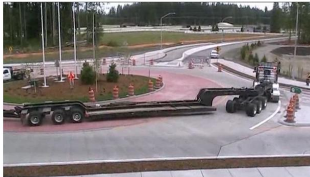
FIGURE 5.15a A Roundabout Designed for a Specific, Local OSOW
