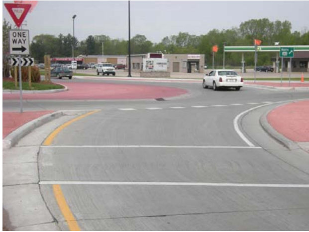
FIGURE 5.12 GE Roundabout in Green Bay, Wisconsin, Modified for OSOW
