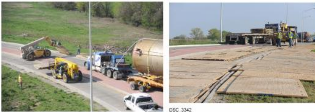
FIGURE 5.32 Two Photos (a-Left, b-Right) of Placing Temporary Mats to Accommodate the 531,000 Pound, 210.5 Foot Long, Round Abatement Tower at the Fredonia, Kansas, Roundabout
