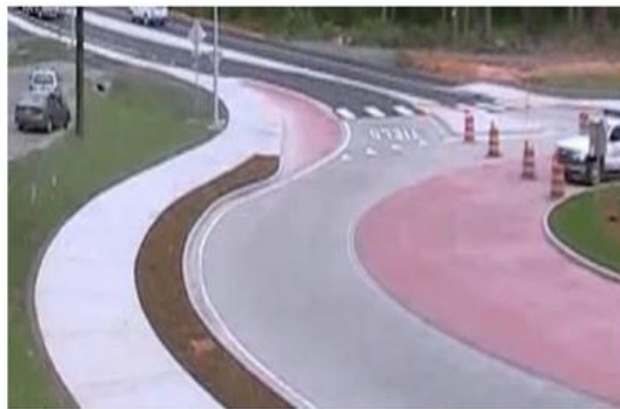
FIGURE 5.15b Entrance of Roundabout in 15a, Designed for a Specific, Local OSOW
