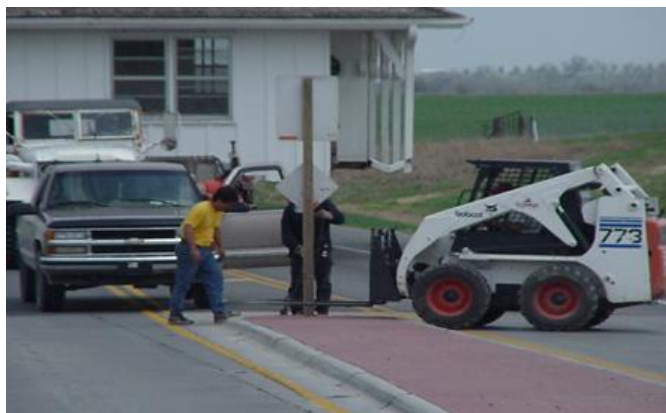
FIGURE 5.3 Removing Signs to Allow a House to Pass through the Paola Roundabout
