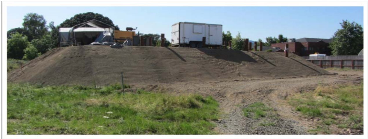
Figure 4.4: Photograph depicting the berm field site pre-testing.
