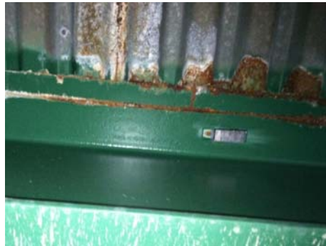
Figure 13: Installed SenSpot strain under the deck of Northwest Branch Bridge on I-495.
