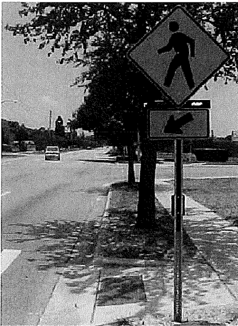
Example of RRFB with W1-2 sign and W16-7p plaque at crosswalk across uncontrolled approach. [Photo courtesy of City of St. Petersburg, Florida]
