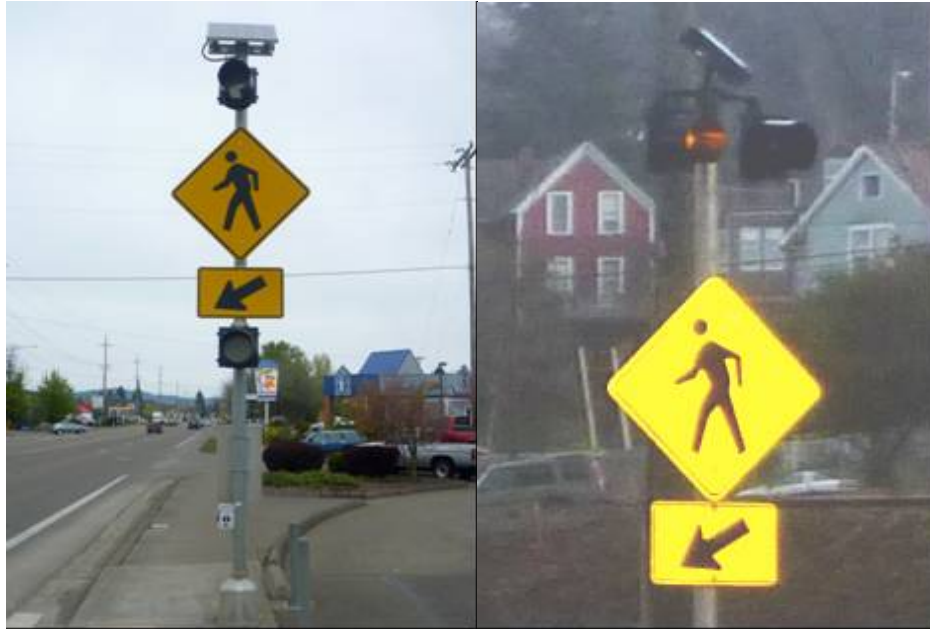
Figure 5.2: Variations of a double yellow beacon (Left: Corvallis, OR; Right: Astoria, OR)
