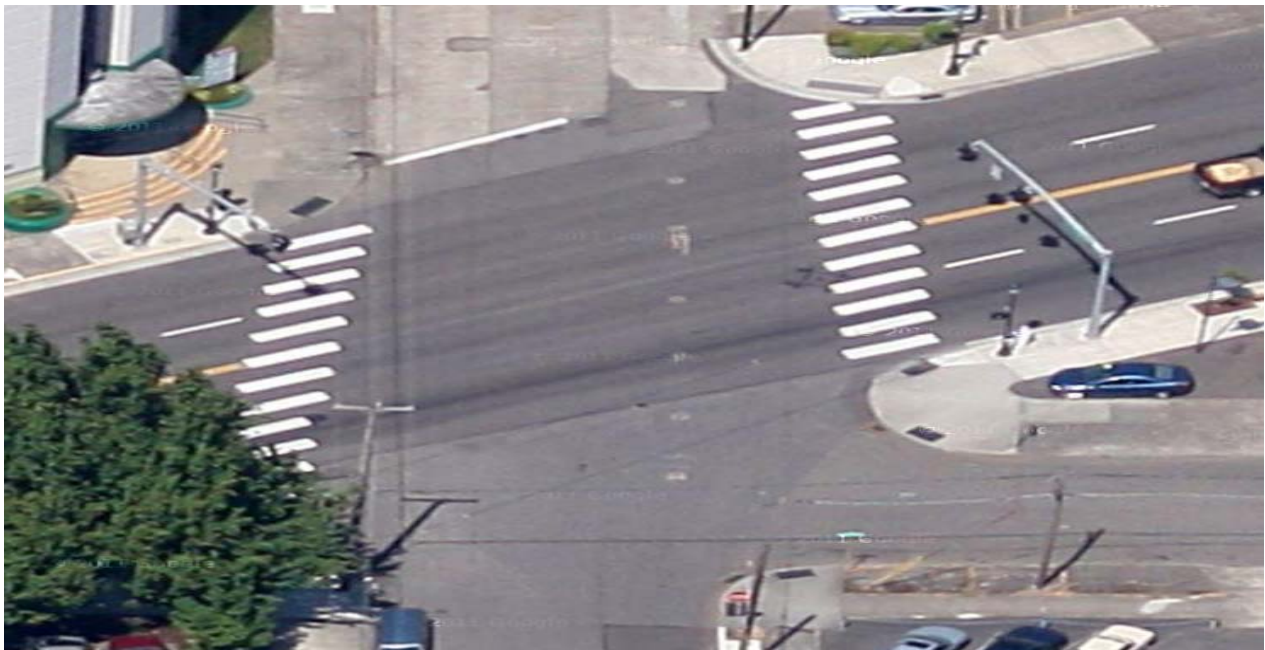
Figure 6.11: Aerial view of PHB at NE Sandy Blvd. and NE 18 th Avenue in Portland, OR
