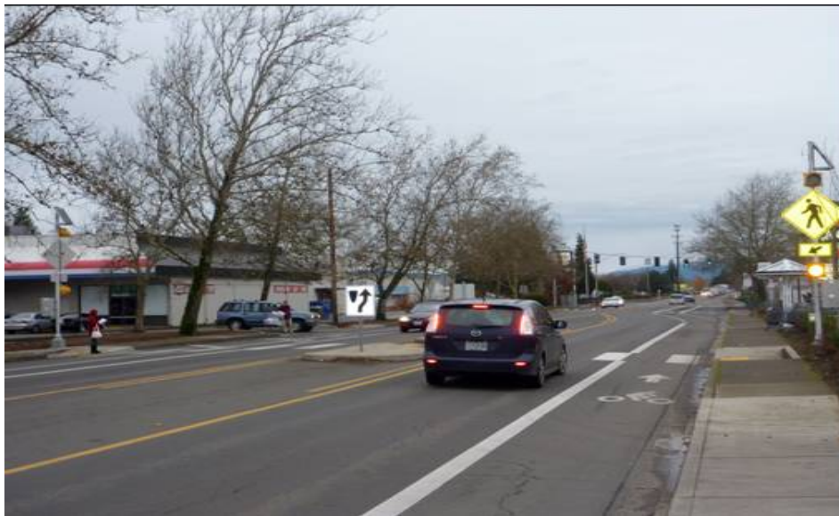
Figure 5.11: Driver perspective of beacon installation on Olympic Street in Springfield
