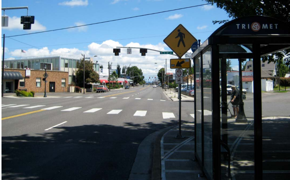
Figure 6.12: PHB installation at NE Sandy Blvd. and NE 18 th Avenue looking east
