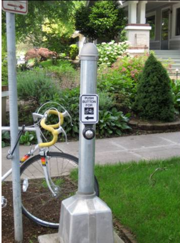
Figure 2.8: Activation button to accommodate bicyclists at a Portland PHB
