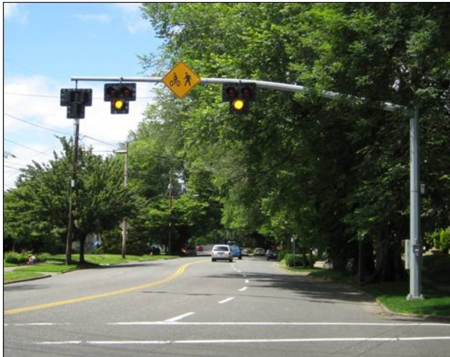
Figure 2.1: PHB installation at NE 41 st Ave and E Burnside St in Portland, Oregon
