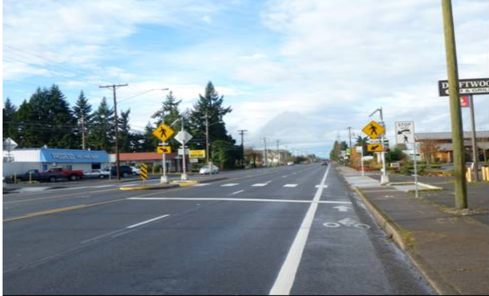
Figure 5.8: Driver perspective of RRFB installation on Main Street in Springfield
