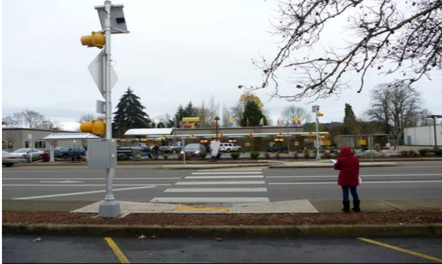
Figure 5.12: Pedestrian perspective of beacon installation on Olympic Street in Springfield
