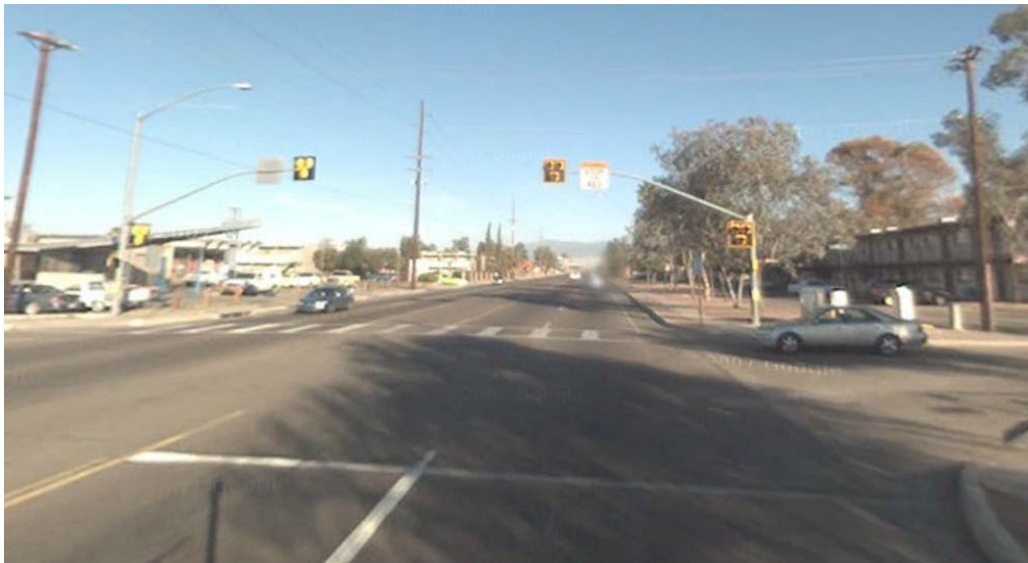
Figure 2.5: Driver perspective at PHB installation in Tucson, AZ
