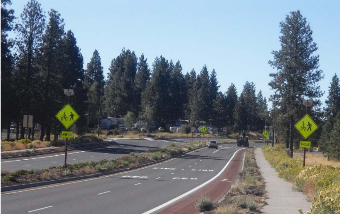
Figure 2.11: RRFB installation at the Reed Lane intersection on the Bend Parkway
