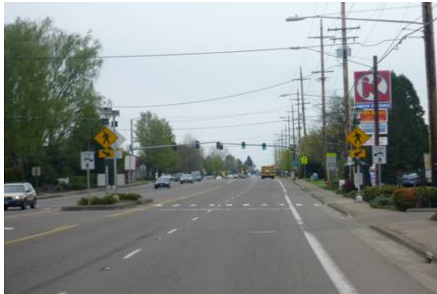
Figure 5.5: Driver view of beacon installation on Highway 99W, Corvallis
