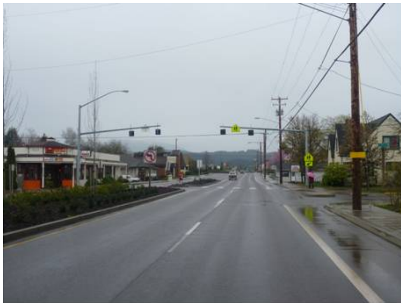
Figure 5.19: Driver perspective of overhead beacon crossing on OR 34 (Main Street) in Philomath
