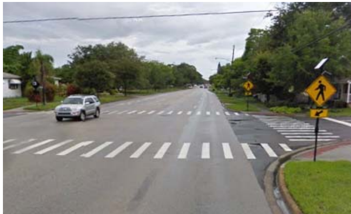
Figure 2.9: RRFBs at an intersection with two crosswalks in St. Petersburg, Florida (Google Maps)
