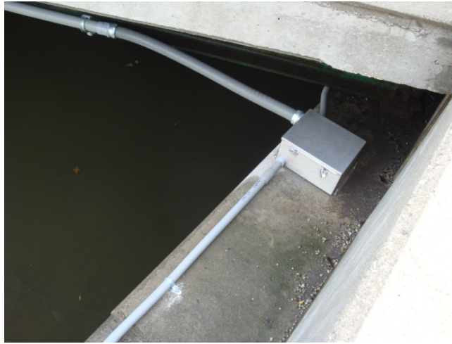
Figure 11. Typical junction box on the abutment.
