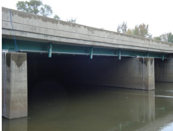
Figure 6. Upstream section of the Salt Creek Bridge.
