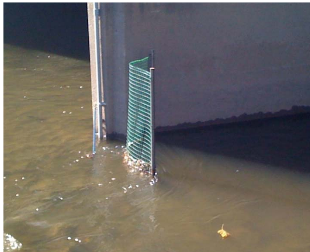
Figure 13. The protective fence system.
