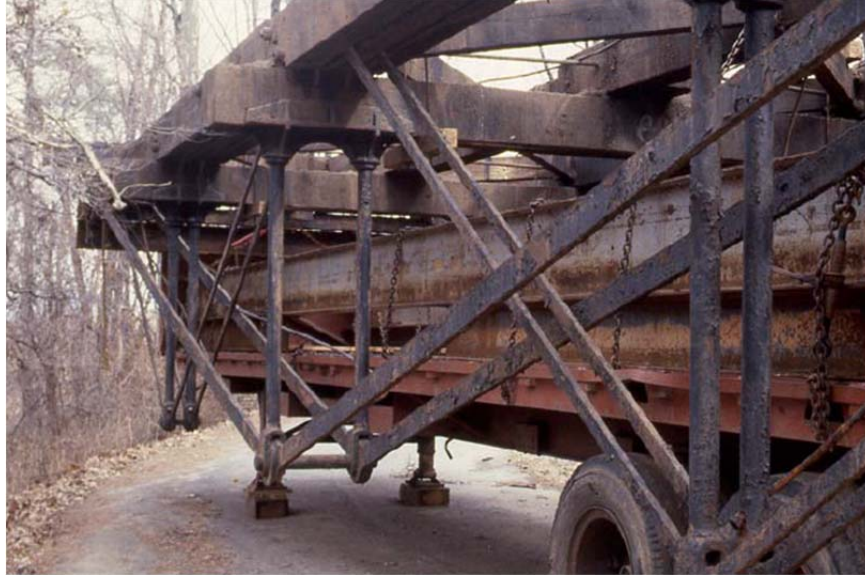
Figure 26. Transportation of Fink truss (VDOT 2006).
