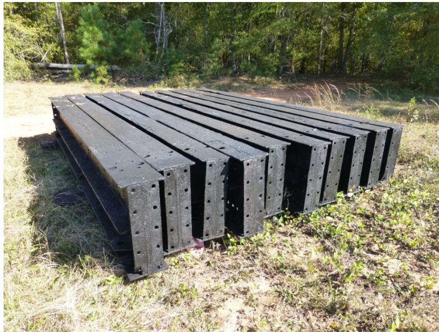
Figure 55. Floor beams in storage at the Griffin-Spalding County airport storage site.
