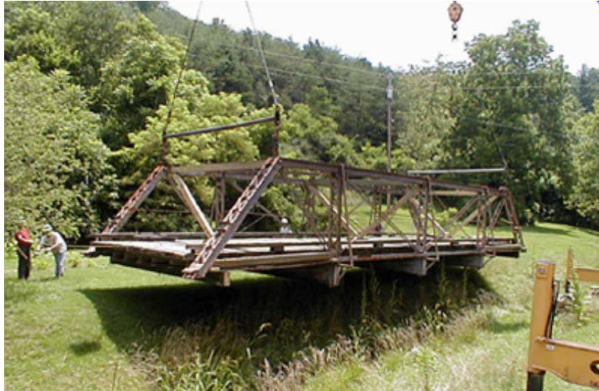
Figure 29. Moving of a pony truss bridge intact (VDOT 2006).
