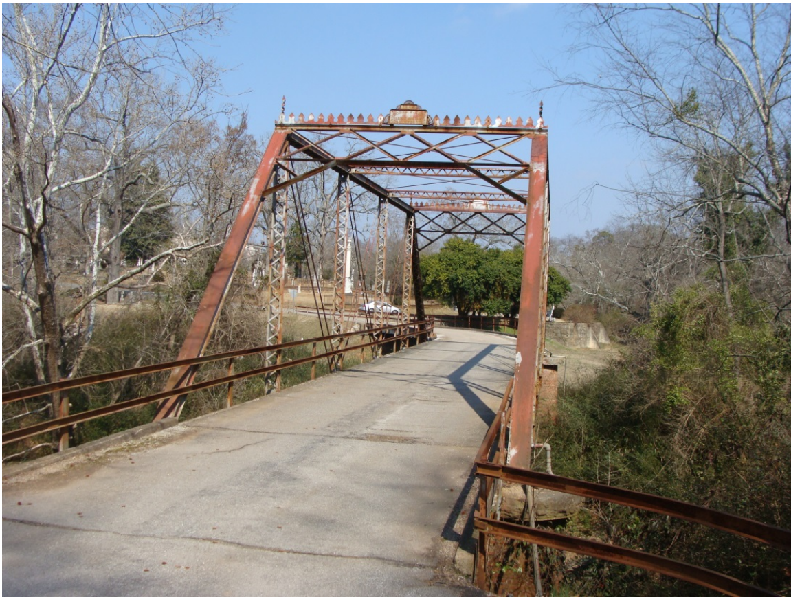
Figure 6. Pratt (pinned) thru truss Clarke County, Bridge 059-9991 (GDOT 2012).
