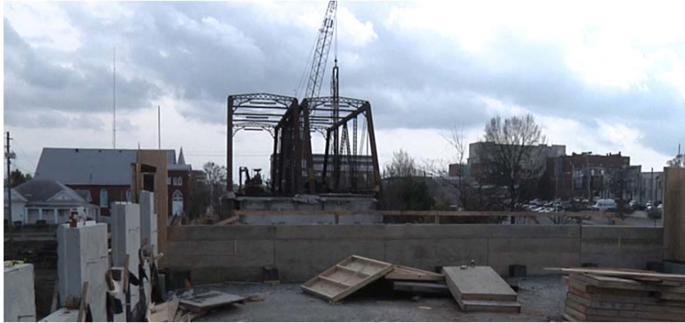
Figure 48. New construction approach spans (Courtesy of Sharman Southall, GDOT).
