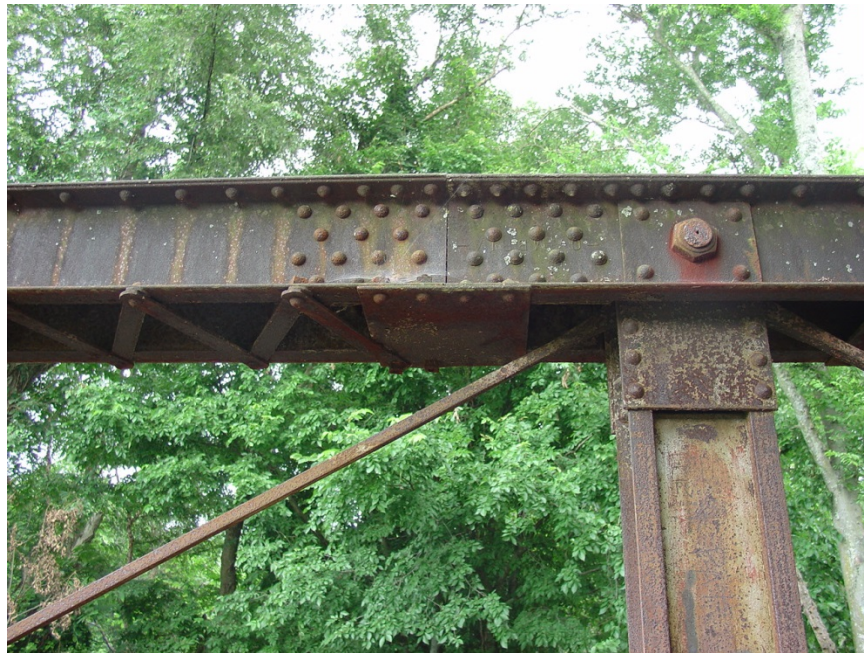
(b) Detail at top chord joint
