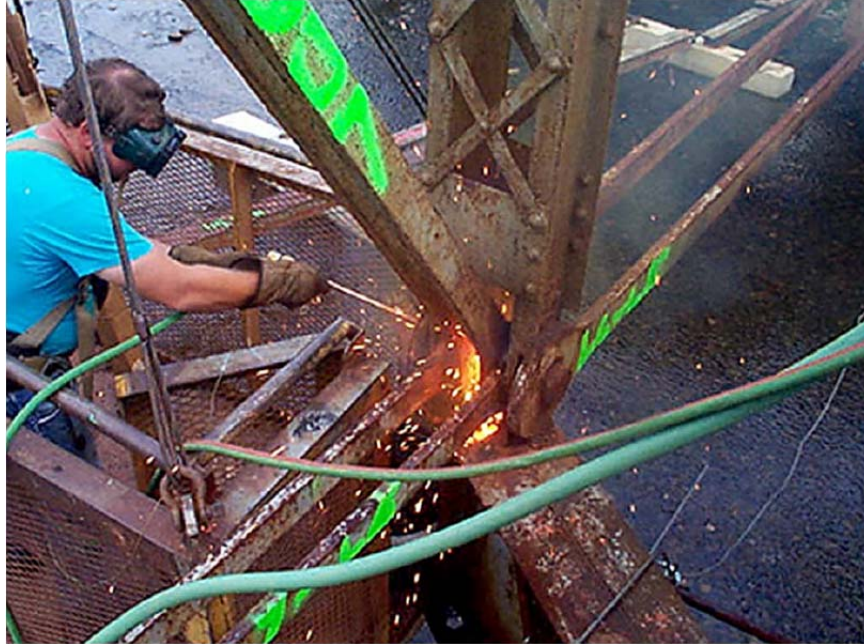
Figure 15. Piercing the center of a pin (VDOT 2006).
