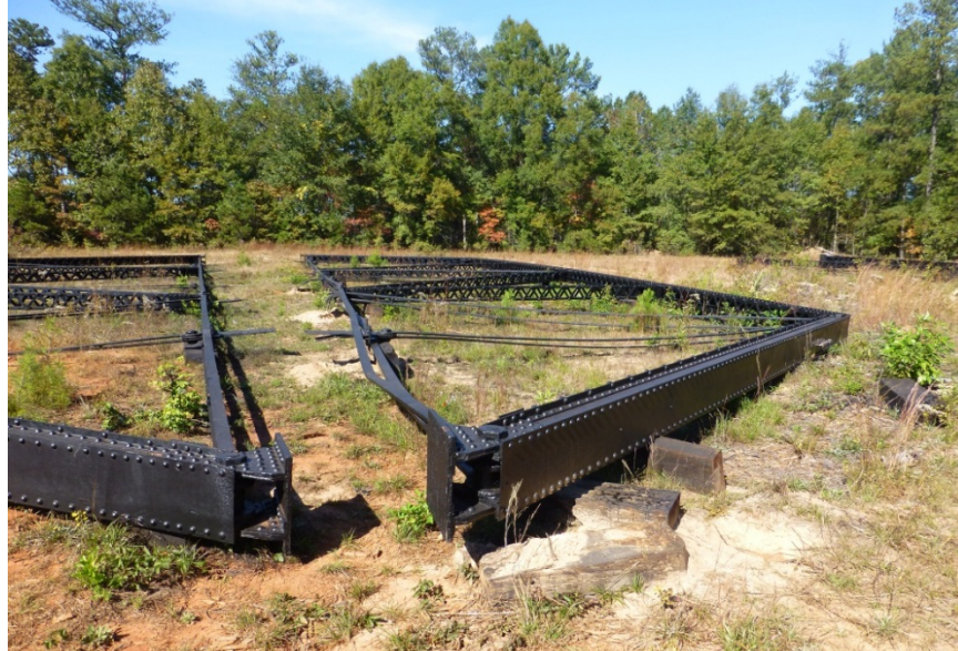
Figure 54. Planar trusses resting on their side on wood blocks at the Griffin-Spalding County airport storage site.
