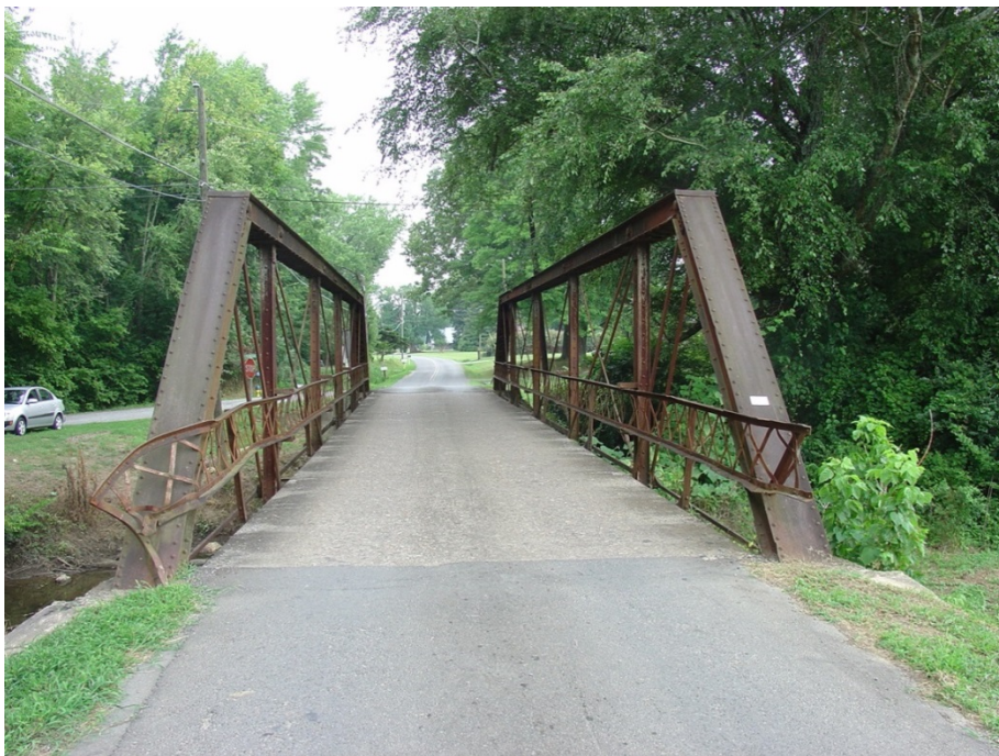
Figure 9. Seventy-nine ft. span Pratt (pinned) pony truss in Murray County, built in 1918 by the Champion Bridge Co., Wilmington, OH, Bridge 213-5007 in the GHBS (GDOT 2012).
