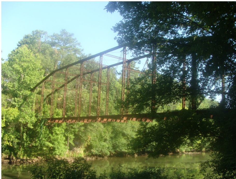
Figure 4. Camelback (pinned) thru truss in Bartow County, Bridge 015-9992 (GDOT 2012).
