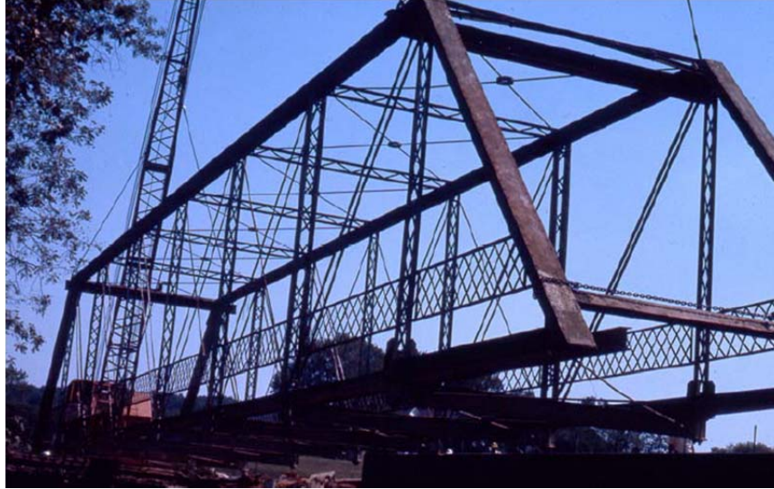
Figure 27. Lifting of a 106 ft. span Pratt truss (VDOT 2006).
