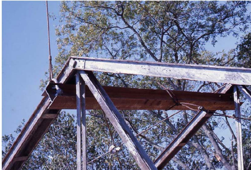
Figure 28. Lifting apparatus at hip joint of 106 ft span Pratt truss (VDOT 2006).
