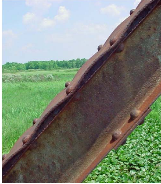
Figure 11. Pack rust (Mesler 2007a)
